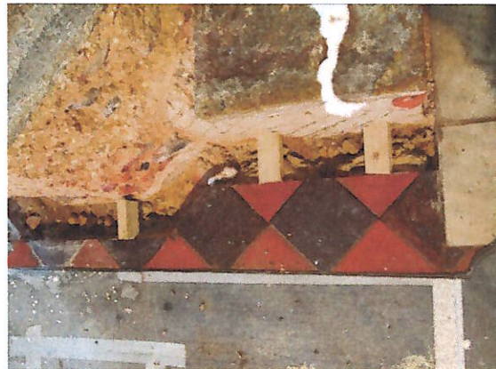
Plates 21 and 22: Re-fixing loose tiles around cut edge
