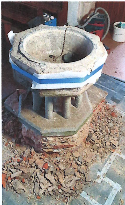
Plate 17: Cement render removal
