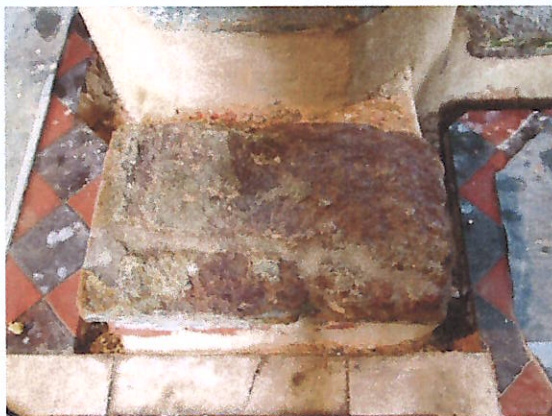
Plate 11: Mortar repair of west step
