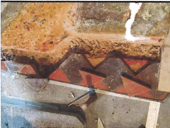
Plates 21 and 22: Re-fixing loose tiles around cut edge
