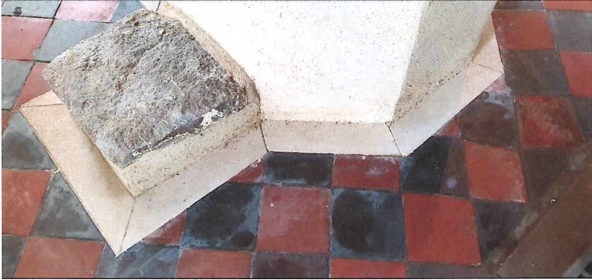
Plate 23: New stone slips installed
