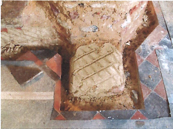
Plate 19: Rebuilding underneath south step
