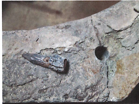
Plate 9: Removal of old iron fixing
