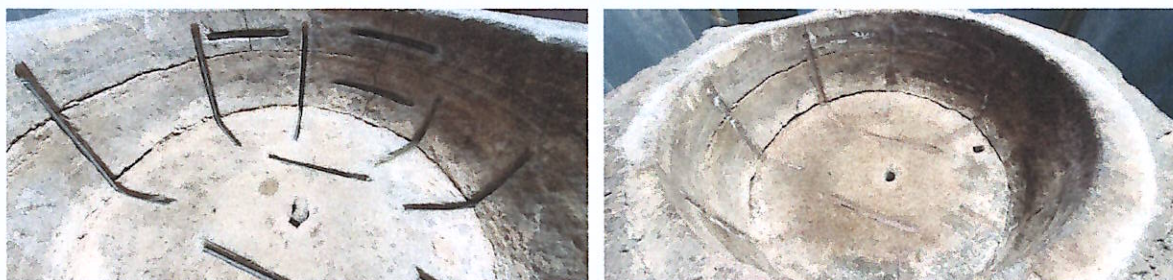
Plates 2 and 3: Dowels before and after being fixed with Hilti HY
