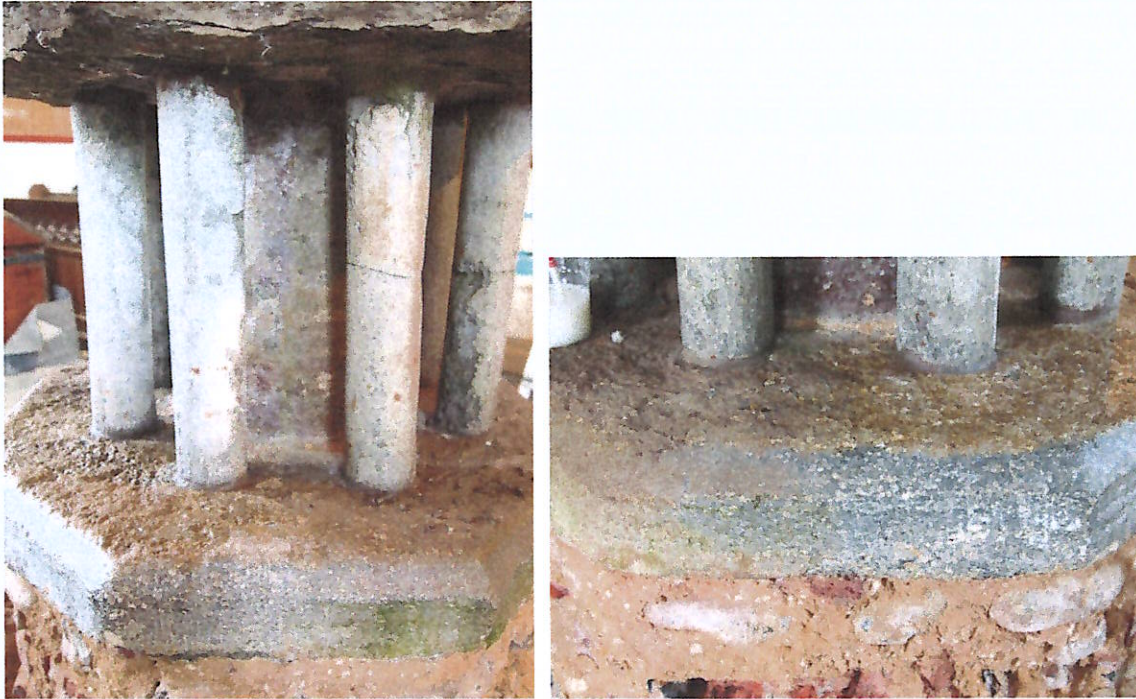
Plates 4 and 5: Cleaning trials of Purbeck marble
