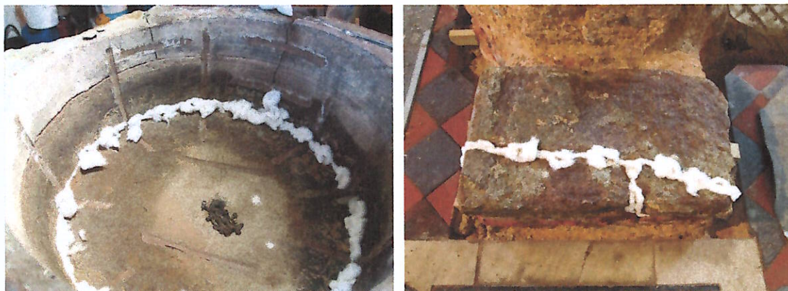
Plates 6 and 7: During grouting of bowl and west step
