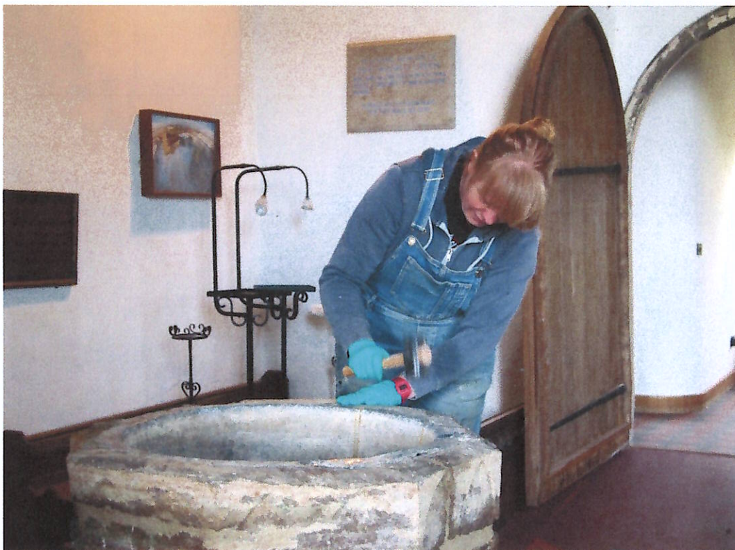
Plate 16: Top of the lead liner being manipulated back into shape
