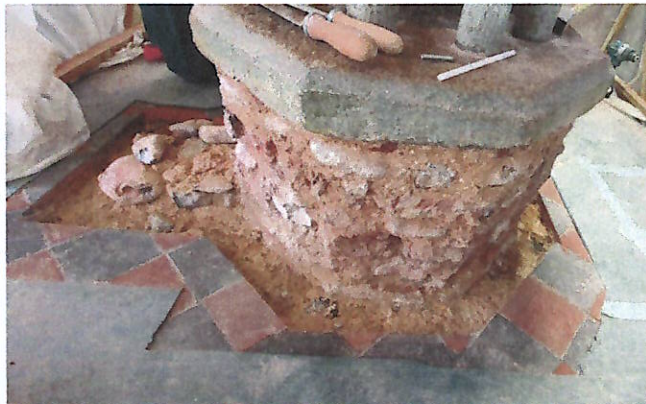
Plate 18: Removal of tiles surrounding plinth
