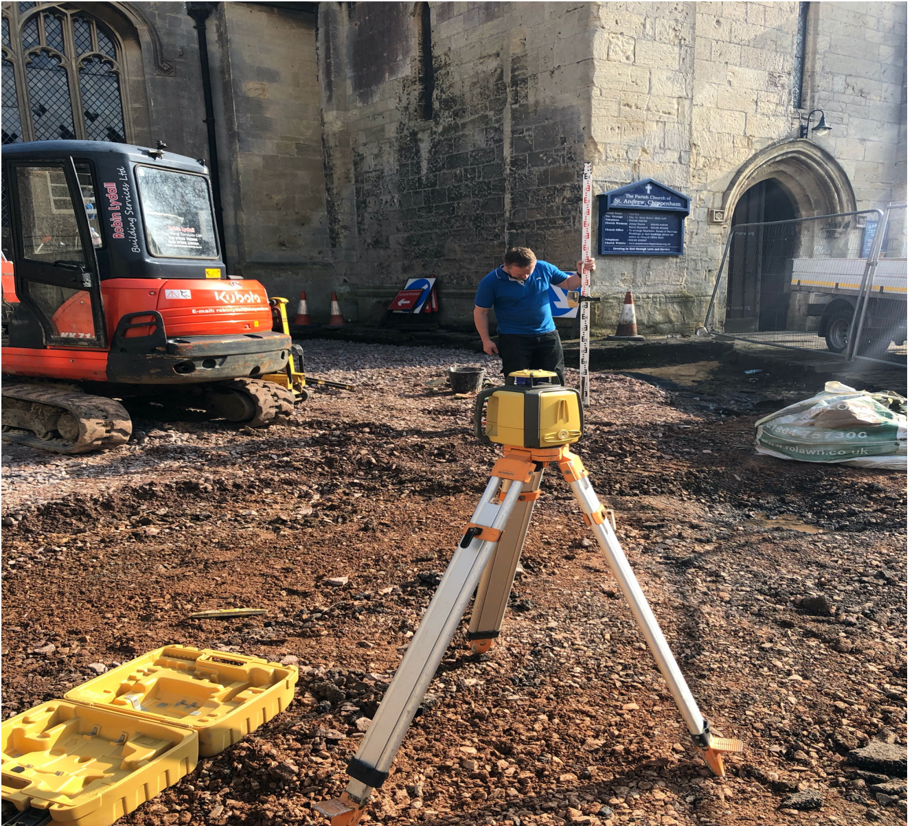
Plate 10 - Leveling in advance of laying Geoblock grid and York paving
