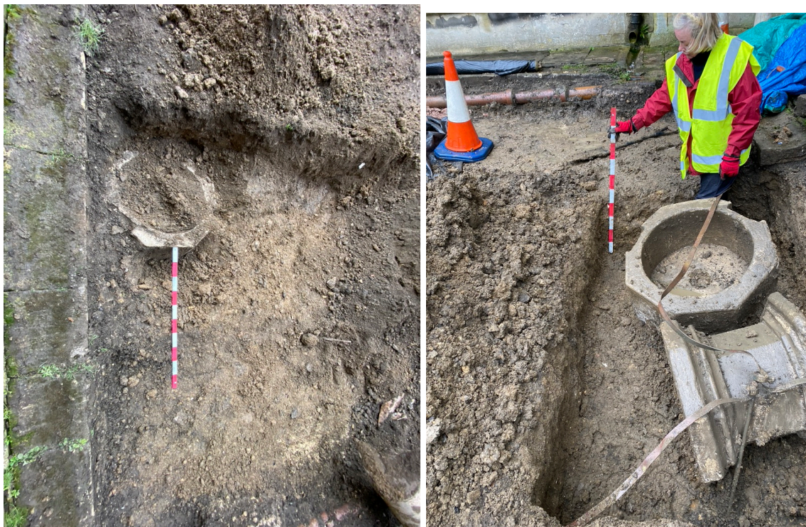
Plate 2. Reburied baptismal font identified just below first scrape of top soil: before and after excavation
