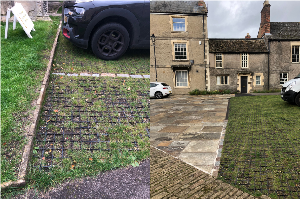
Plate 11-14 Detail of finish above and below: Geoblock with grass sown, reused stone edging and cobbling
