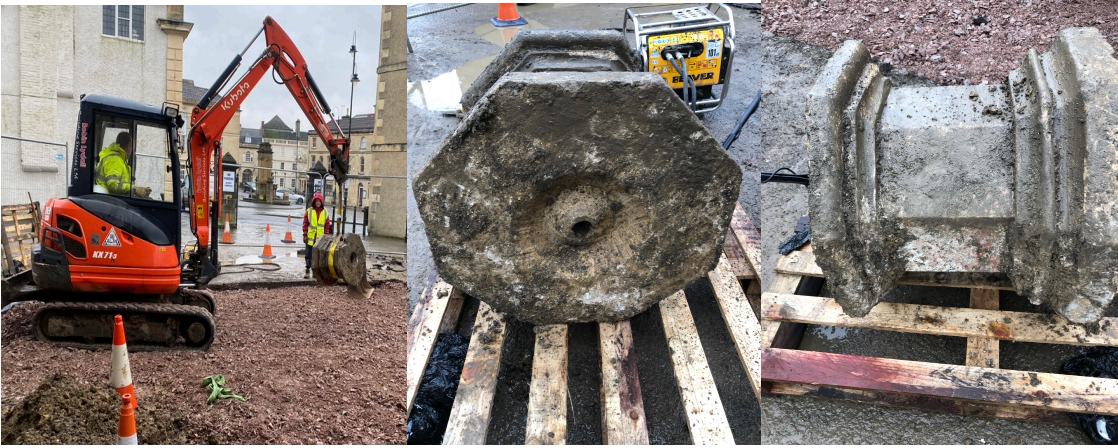
Plate 5-7: lifting font off site onto pallets for drying
