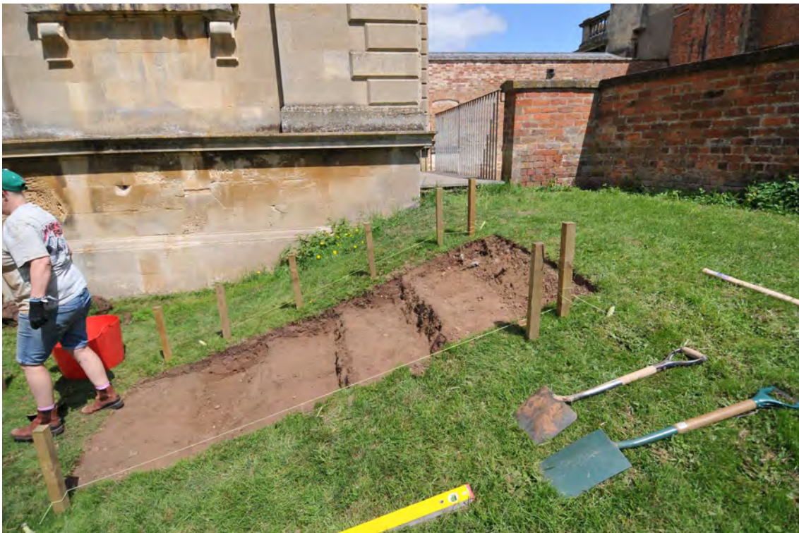
View of excavation for new steps facing north
