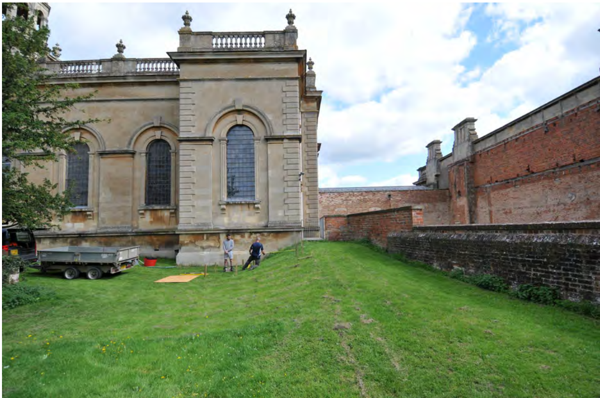
Location of new steps on flank of fire exit ramp (view facing north)
