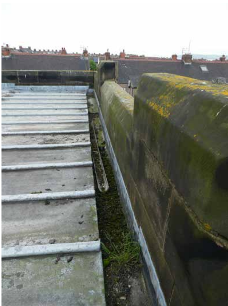
Failures in the lead include splits at the bottom of the rolls (highlighted). These have been temporarily repaired with mastic in the past.
