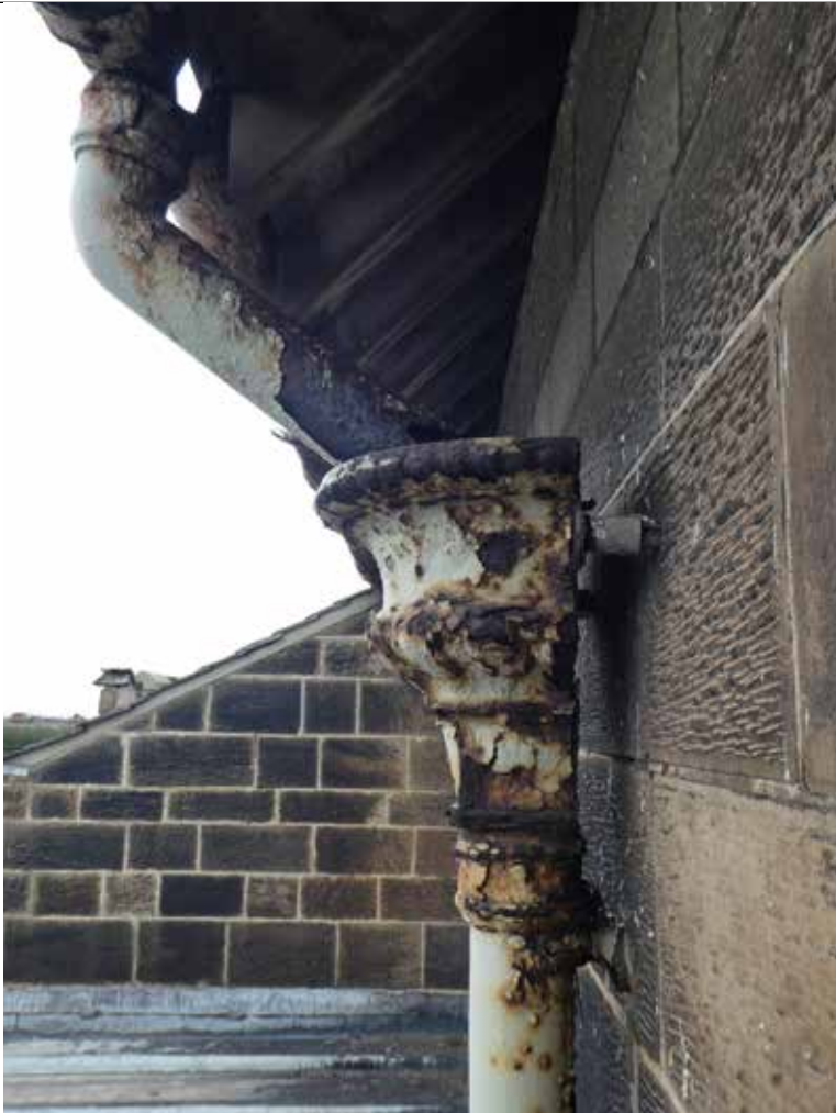
Some sections of the existing rainwater goods at high level were in a poor condition. While the gutters were replaced with new cast iron, the existing hoppers and downpipes were salvaged and kept.
