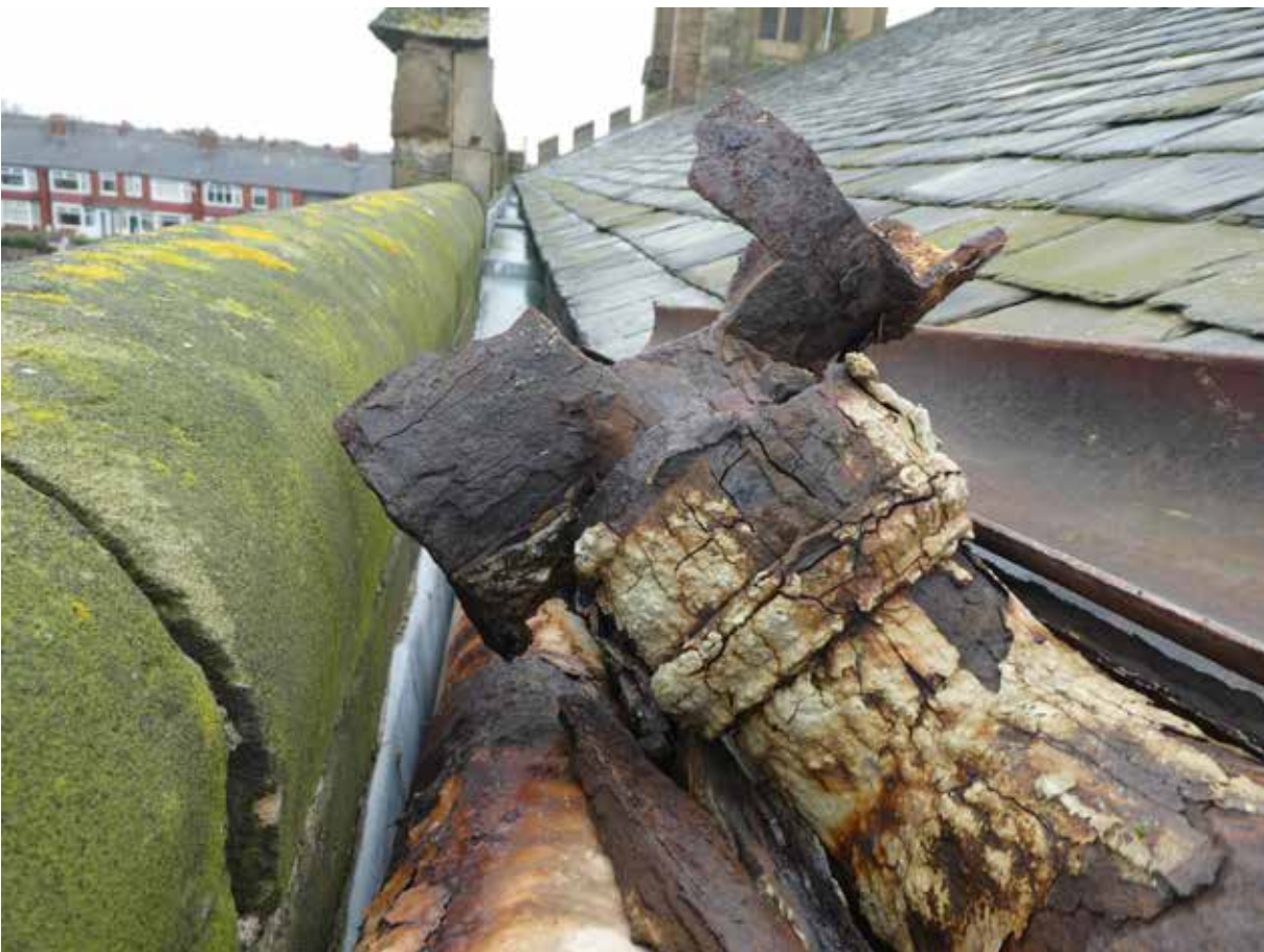
Some sections of the existing rainwater goods at high level were in a poor condition. While the gutters were replaced with new cast iron, the existing hoppers and downpipes were salvaged and kept.
