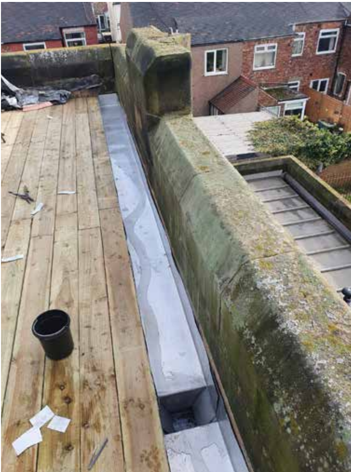
Testing the new stainless steel gutter.
