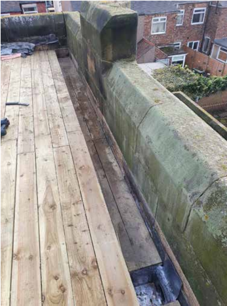
New gutter boards and lead sump in place.
