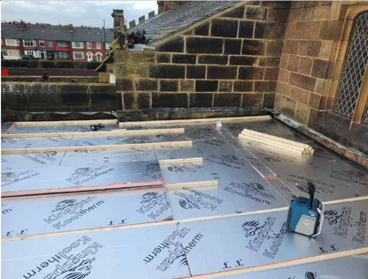
Installation of the insulation layer.
