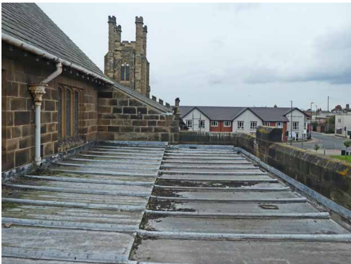
The existing lead roof on south side of Chancel (looking west).
