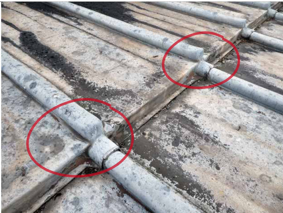
Failures in the lead include splits at the bottom of the rolls (highlighted). These have been temporarily repaired with mastic in the past.
