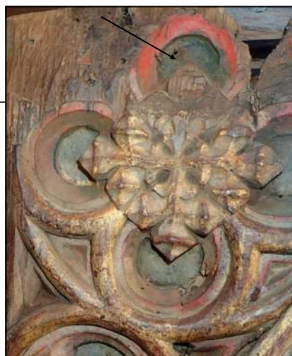
Location of sample 11 (see arrow above), taken from the blue background of a quatrefoil in a spandrel on Bay 5 arcade.
