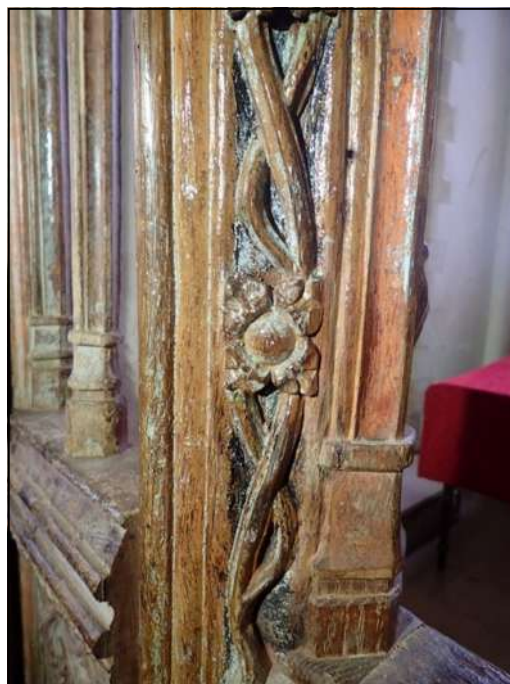
North screen arcade. Above left, view and location of sample 6 (see arrow). Above right, detail of carved post, north screen, showing pale blue overpaint which in places is flaking. The appearance of these surfaces would be considerably improved if the overpaint were removed.
