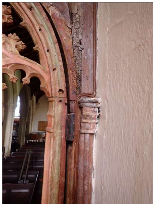
East face detail showing how wall coatings butt against the screen.
