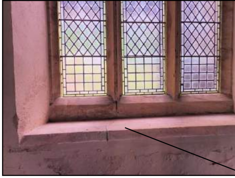
Cracks under window WS3 (above interior, below exterior) will be contributing to damp on this wall
