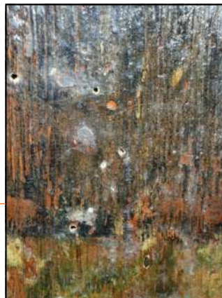
Details of active beetle attack on south screen figure panel.
