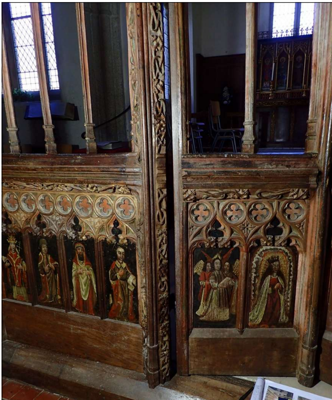
Bay 4 and the north side of Bay 5 chancel screen doors, which depict the Choir of Angels and the Blessed Virgin. Much of the upper tracery carving here is original with extensive polychromy., as is also found on the foliate trail around the doorway.
