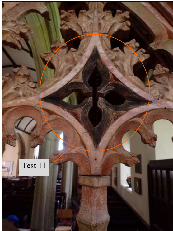
East face, Bay 1, showing extensive colour survives here too, visible clearly after wetting-out tests. Further tests were followed by the application of Paraloid B72 in Acetone/IMS, where poorly bound paint needed isolating before varnishing
