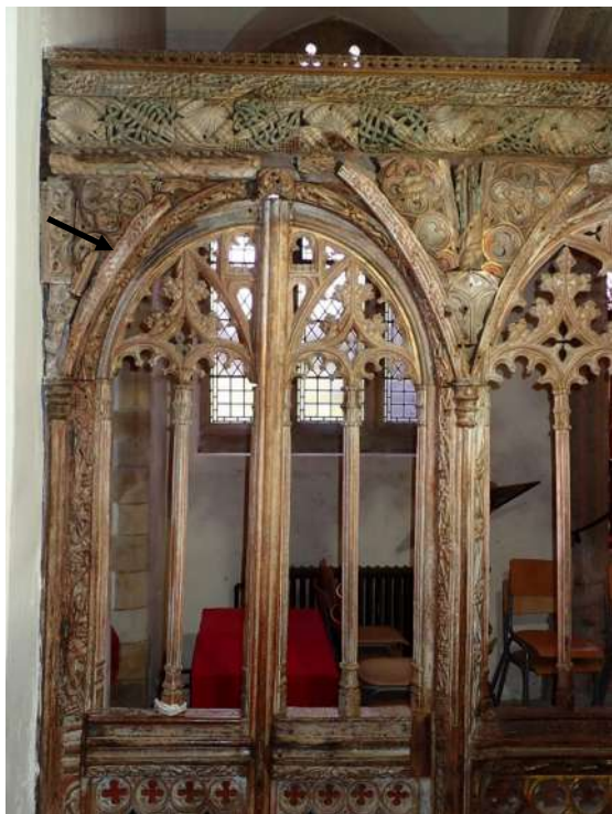
North screen arcade. Above left, view and location of sample 6 (see arrow). Above right, detail of carved post, north screen, showing pale blue overpaint which in places is flaking. The appearance of these surfaces would be considerably improved if the overpaint were removed.
