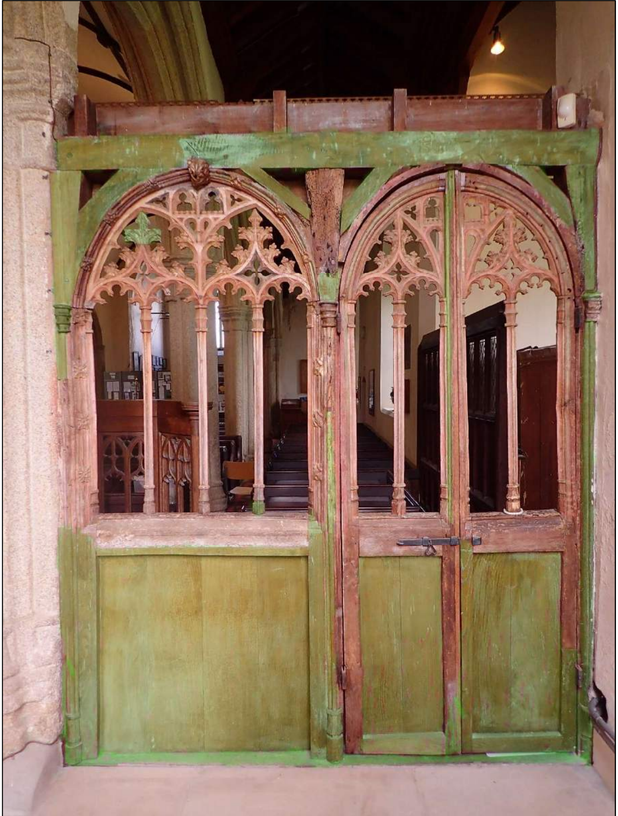
North Screen, East Face
