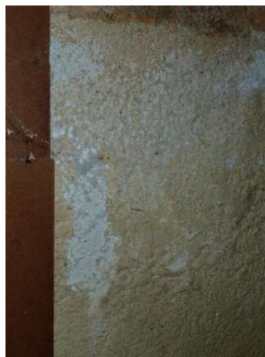
The window in the east wall has been blocked and dampness in the wall is causing adjacent paint to detach in sheets (see details above and below).
