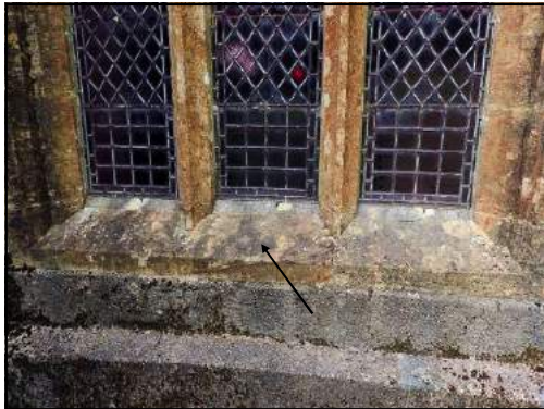
Cracks under window WS3 (above interior, below exterior) will be contributing to damp on this wall
