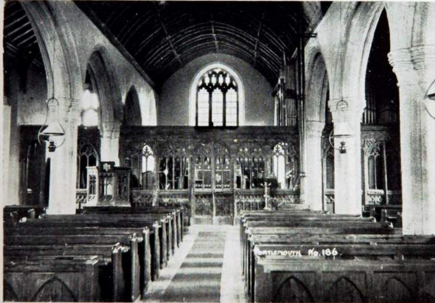
BEFORE THE 1936 RESTORATION.
