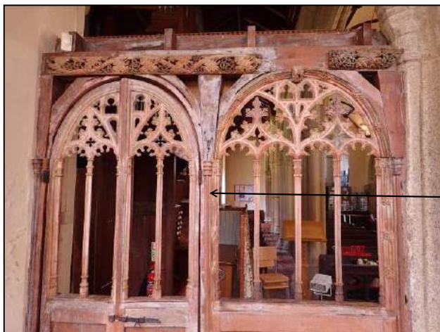
The east face of Bays 8 and 9, south screen.
