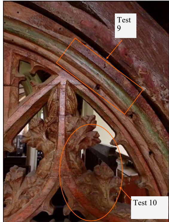
East face, Bay 1, showing extensive colour survives here too, visible clearly after wetting-out tests. Further tests were followed by the application of Paraloid B72 in Acetone/IMS, where poorly bound paint needed isolating before varnishing
