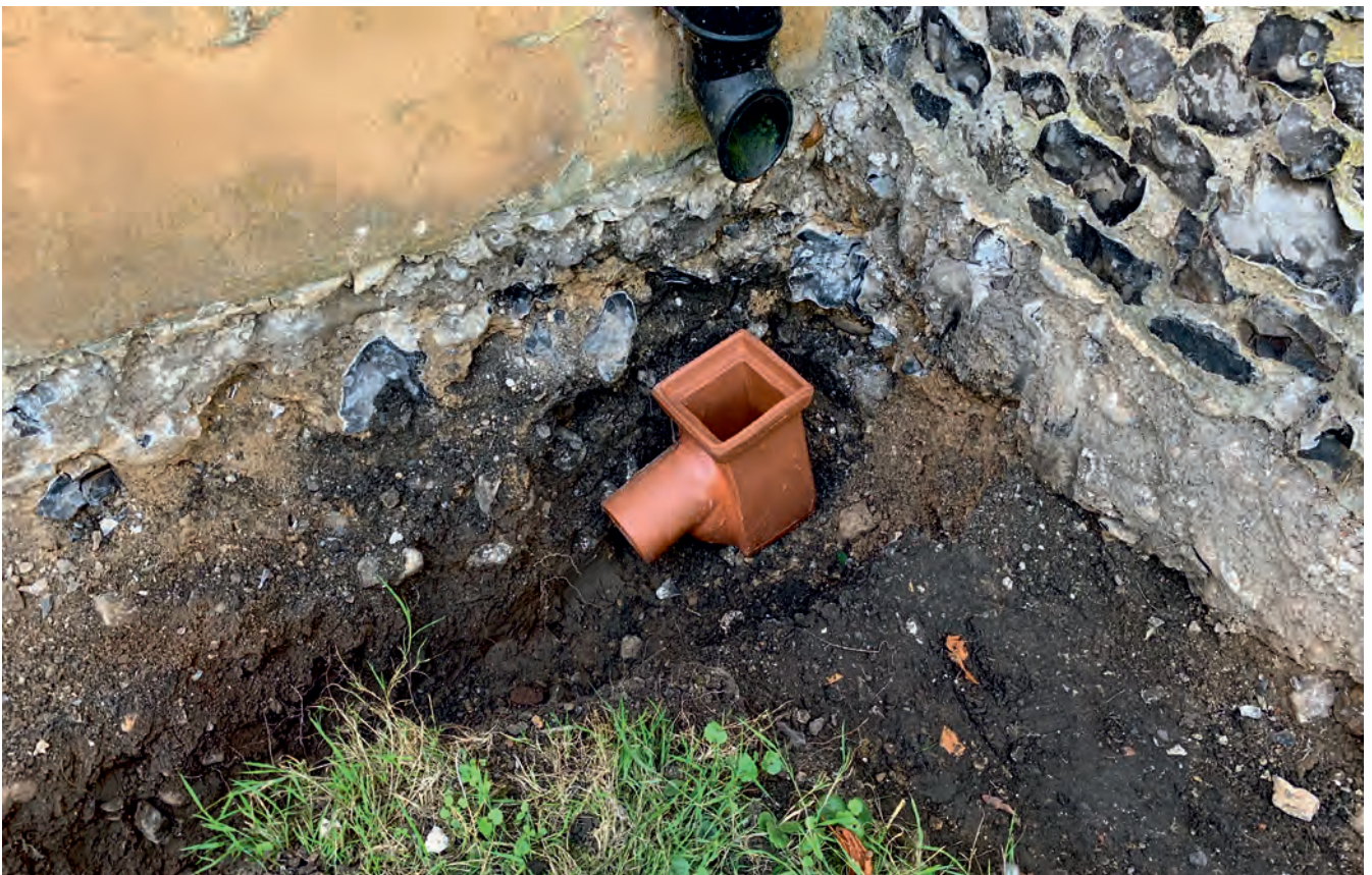
Plate 6. View of the junction between the north aisle's east wall and the chancel's north wall exposed in drainage trench DT2 showing the junction of the two separate medieval period foundations.
