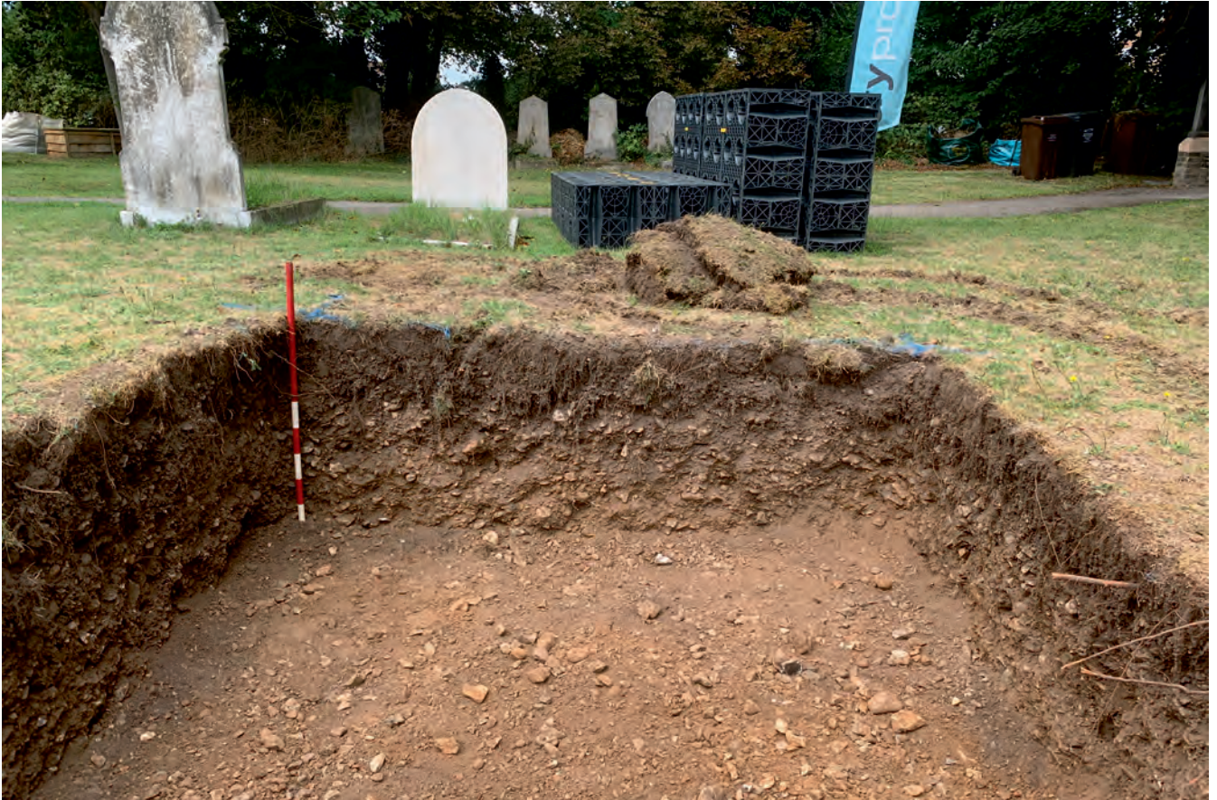
Plate 7. View looking west at the western section of soakaway position S1 showing graveyard deposits over natural gravel geology and sealed by topsoil.
