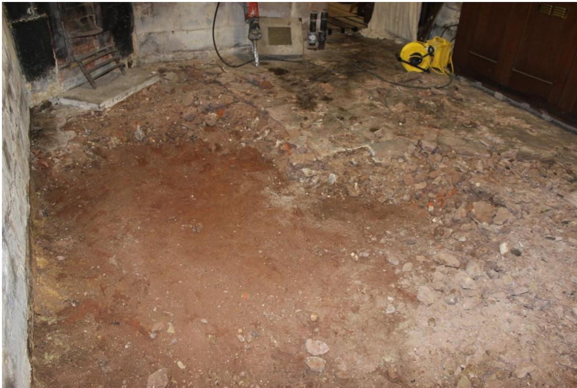
**Plate 2: Breaking up the concrete floor**
