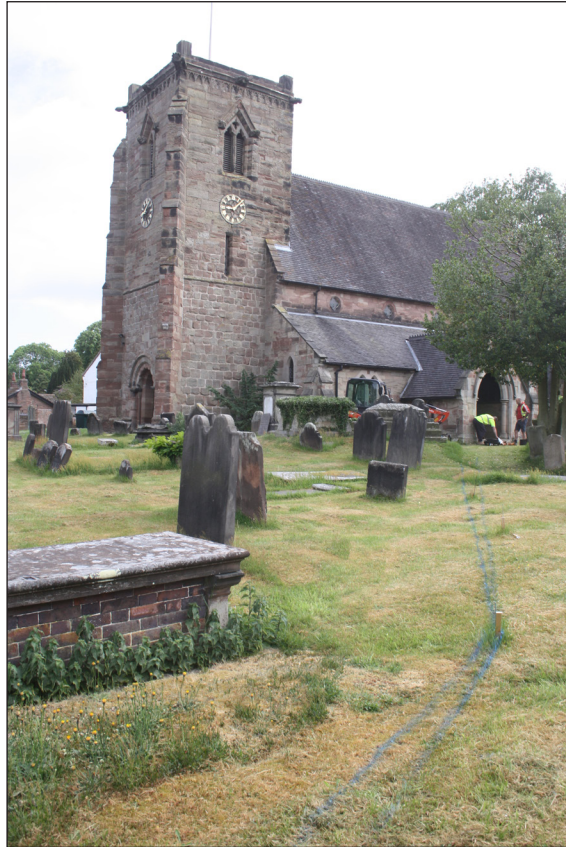
Plate 1. Churchyard of St Mary showing course of pipe trench, looking NE from boundary.
