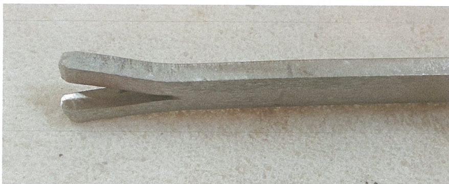
Plate 14: detail of the fishtail at the end of all restraining cramps fixed into wall
