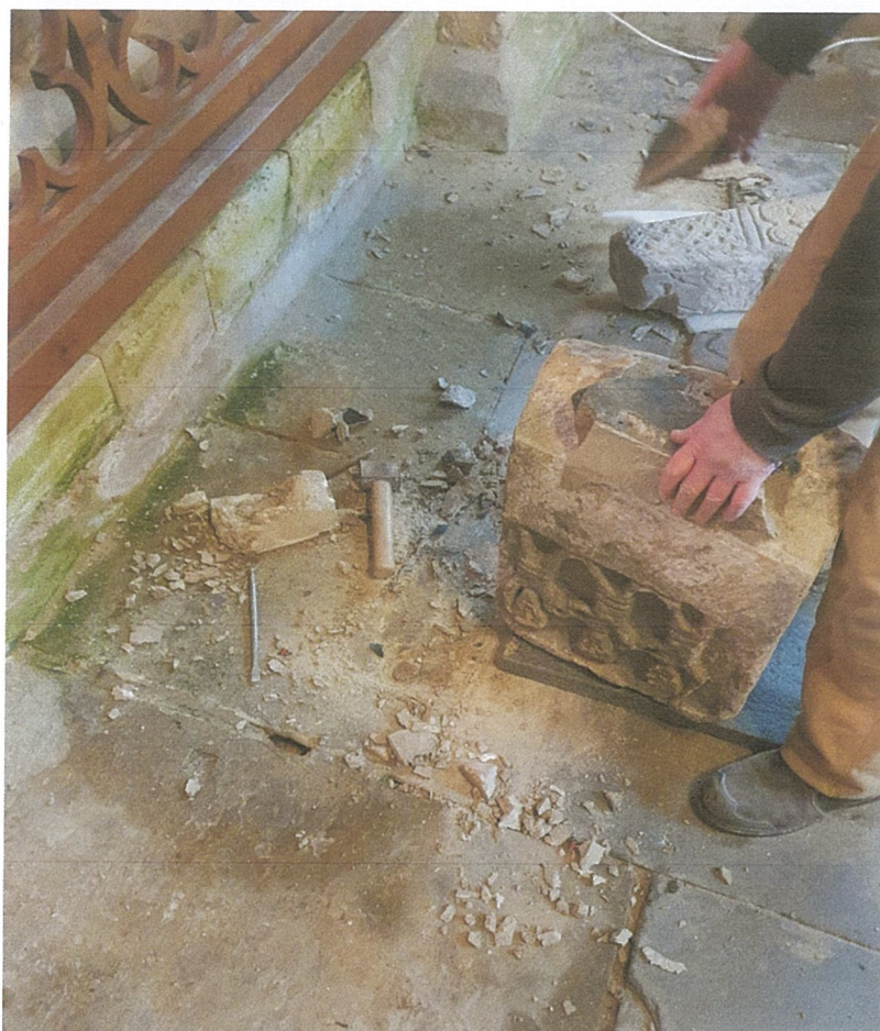
Plate 6: During the process of removing the stone cross fragments from the flag floors.
