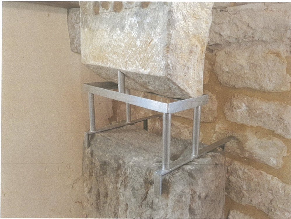
Plate 9: The frame for fragments 1 & 2. Note the additional support for fragment 2
