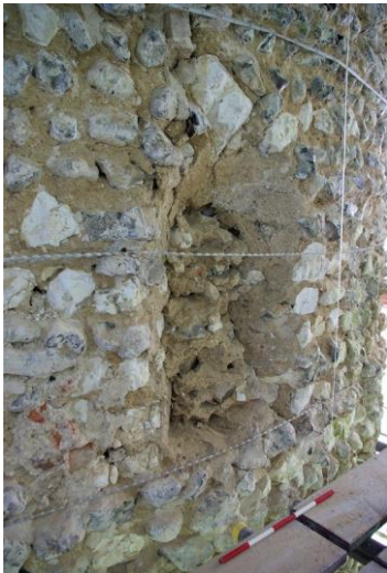
Plate 37: Window [17], blocking mostly removed, looking SE 0.5m scale
