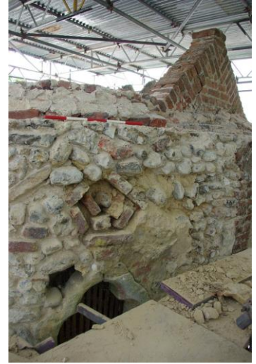
Plate 49: N gable and pentagonal opening [70] above cusped opening [9], looking SW, 0.5m scale
