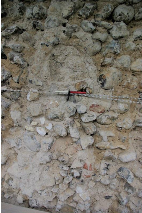
Plate 43: Window [24], blocked and with surrounding repairs, looking N, 0. 2m scale
