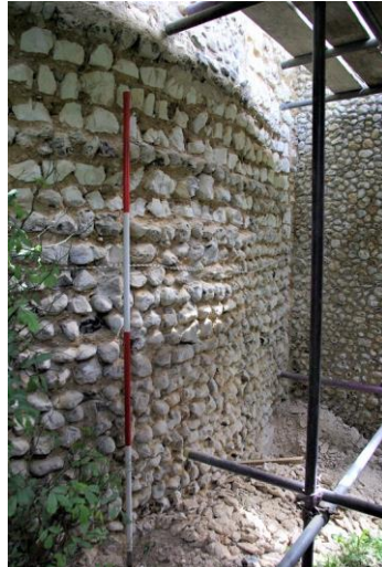
Plate 23: Tower S side, lower stage [33], ground level, (chalk courses at top), looking E, 2m scale
