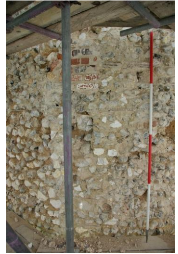
Plate 33: SW side, central stage, repair [23] with different wall fabric to either side, looking NE, 2m scale
