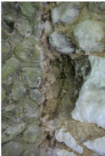
Plate 28: Tower abutting former nave wall (detail), Victorian wall to left, looking SE
