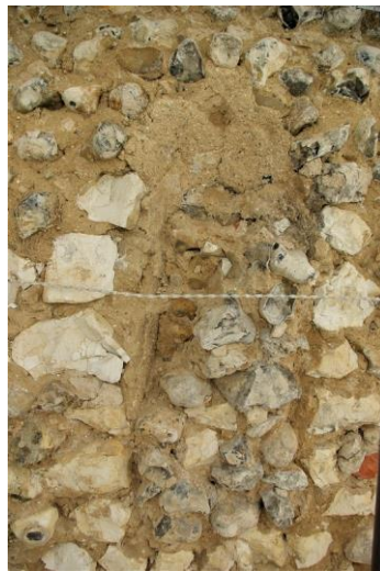
Plate 41: Window [21], looking E
