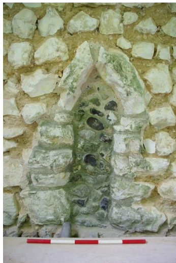
Plate 29: N side, window [30], looking S, 0.5m scale
