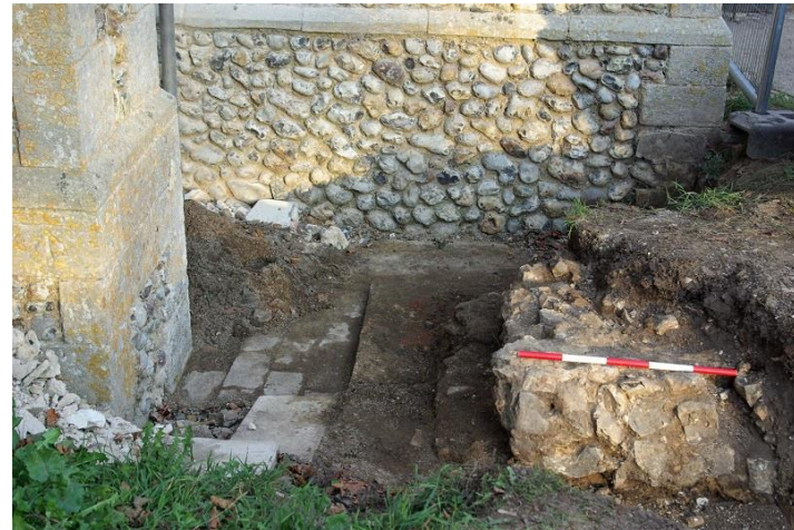
Plate 16: Trench 53, wall footing [58], looking E, 0.5m scale
