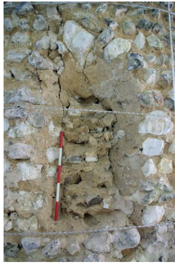
Plate 38: Window [17], blocking mostly removed, looking S 0.5m scale
