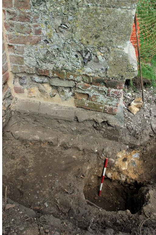
Plate 13: Trench 39, footing at chancel SE buttress, looking E, 0.5m scale
