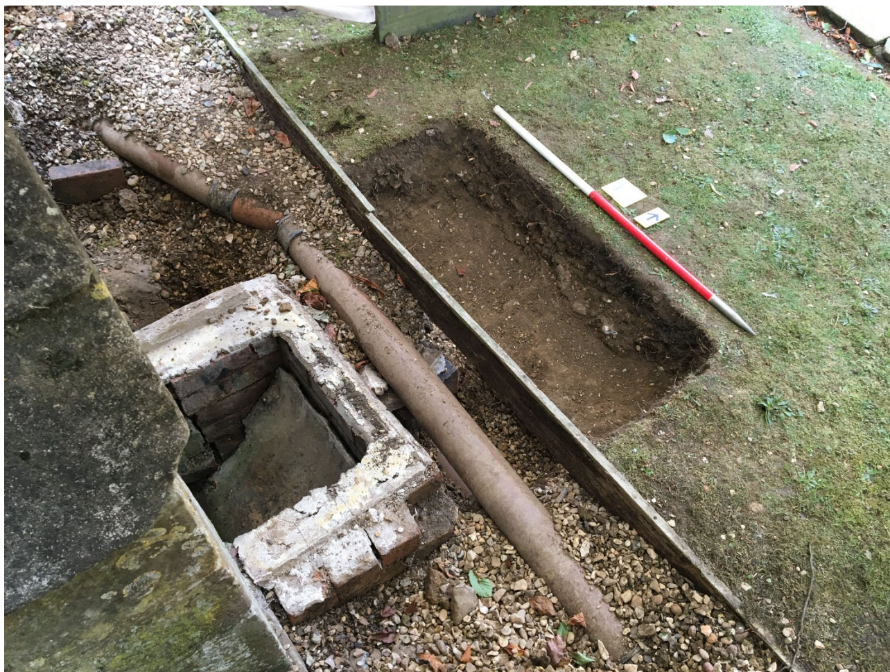
Figure 8: The coal chute and drain dug into the burial soil in front of the original crypt entrance, looking north-west.
