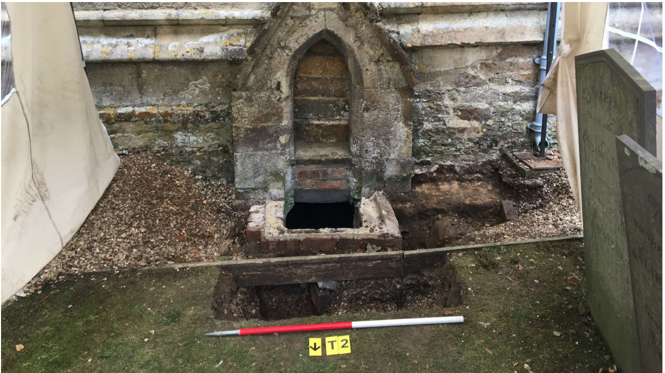
Figure 7: Test-pit 2 in front of the original entrance to the crypt, looking south.
