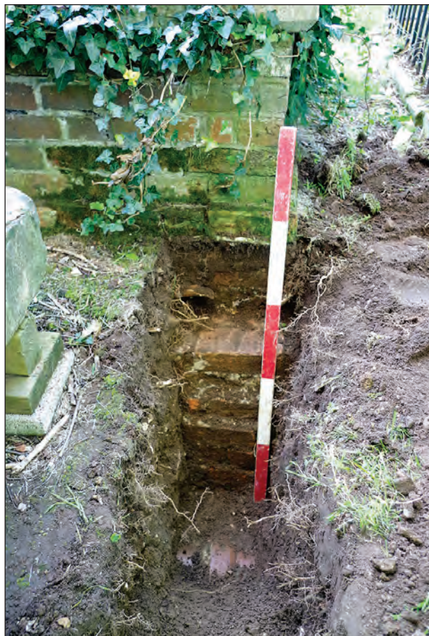
Plate 2: North facing section of Test Pit 1, detailing brick vault. Scale is 1 m
