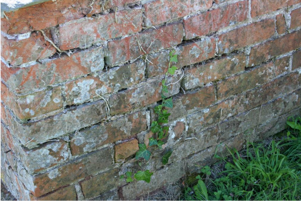
7 and 8. ivy growth and open joints affecting the Roll tomb
