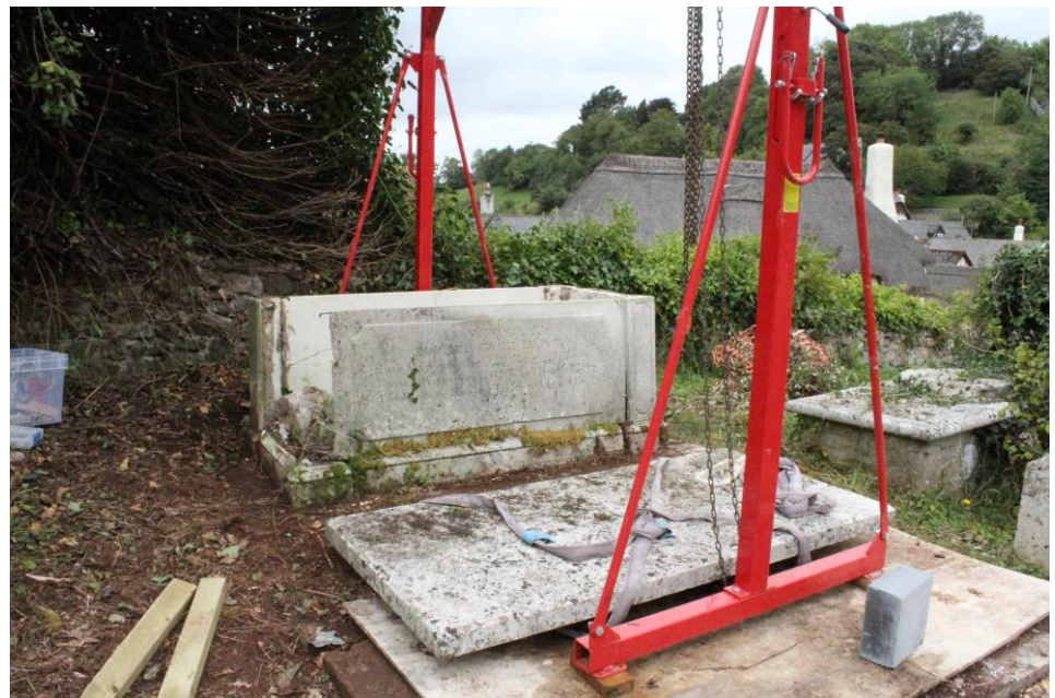
12. below; top slab removed and place on moving skates
