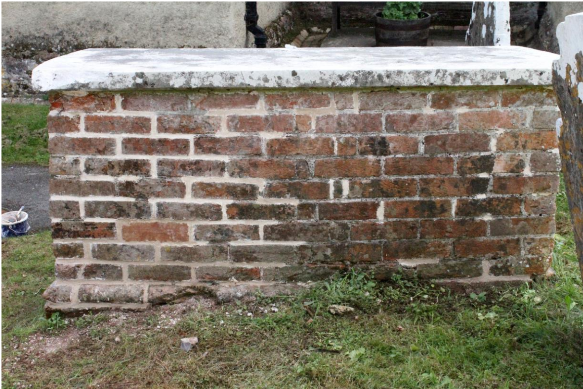
30. Below, Mary Roll monument complete, view from the south
