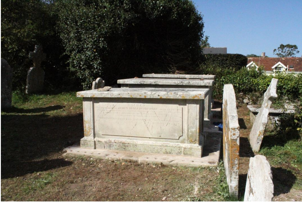
25. Above, the three stone monuments when work was complete
