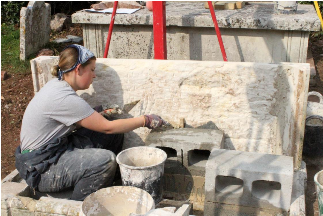
23. above, pointing work in progress
