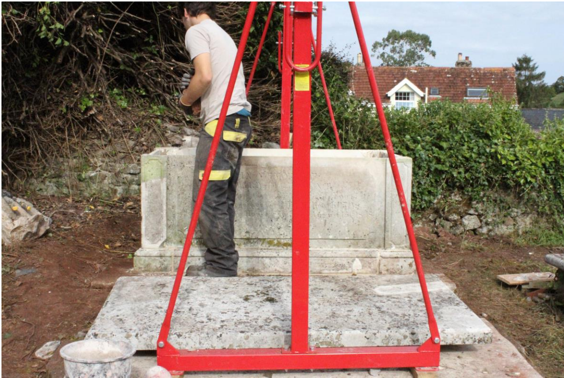
21. Above, re-erection in progress
