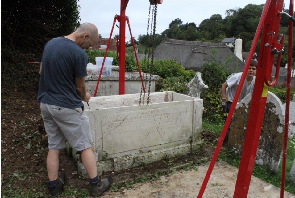
11 Above; lifting gantry in use
