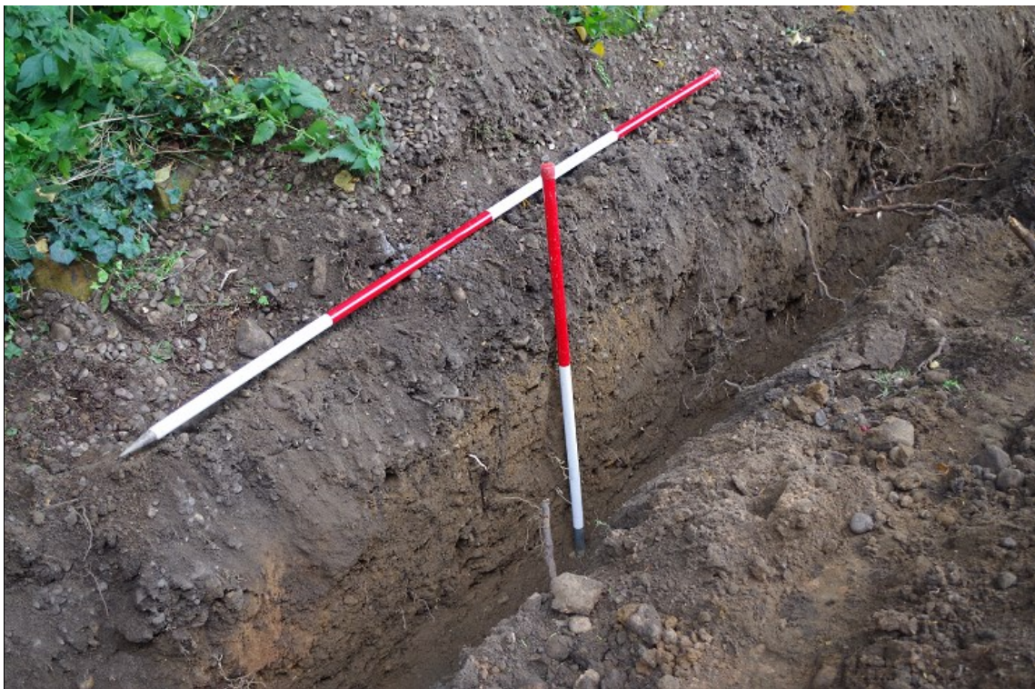
Photo 6. Detail shot showing typical deposit sequence within service trench, looking N.
