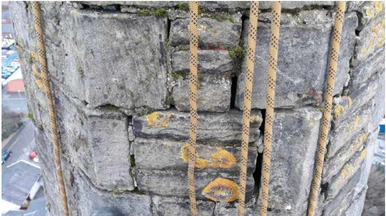
Pointing West face
