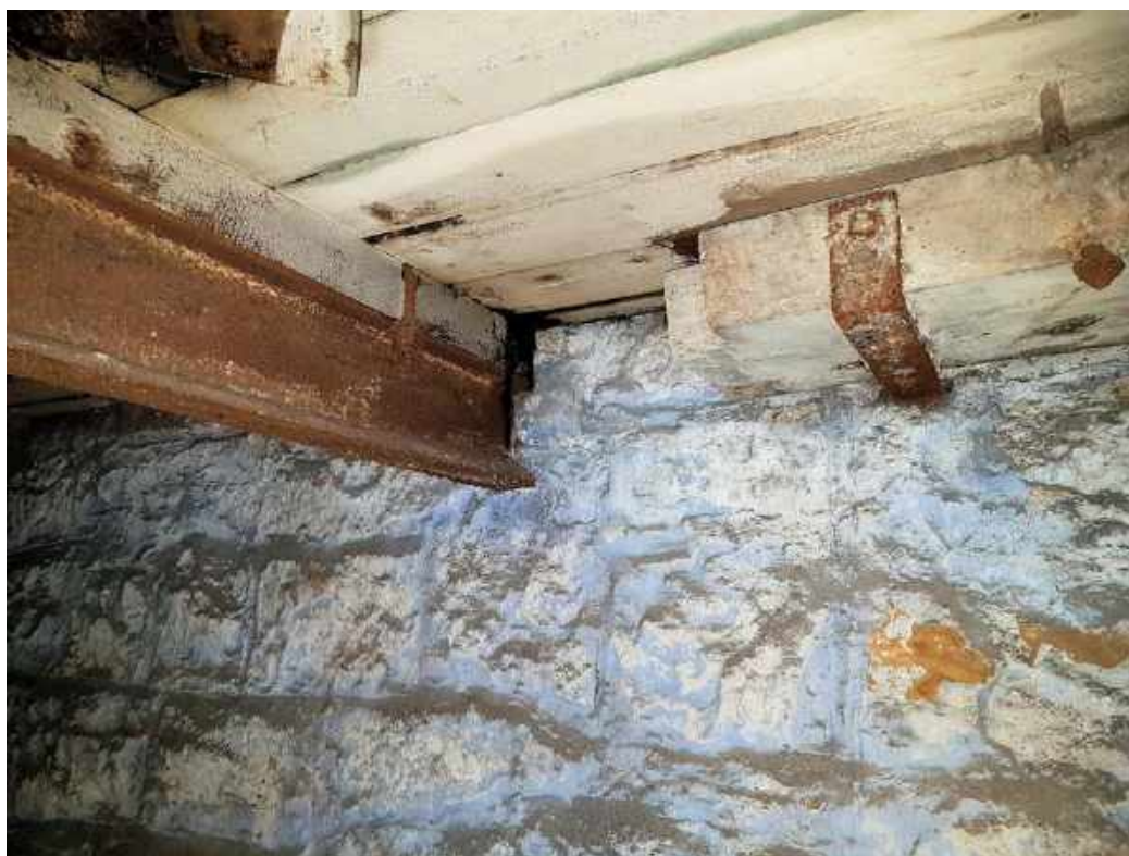
3 rd floor supports
