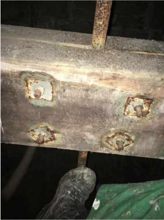
Boards clamped around HD rod
