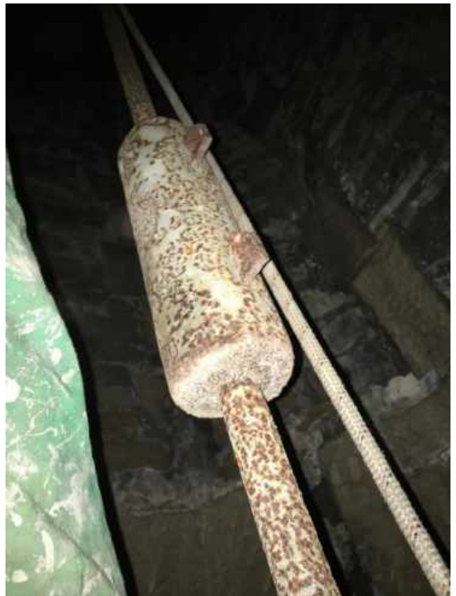
Holding down rod coupling
