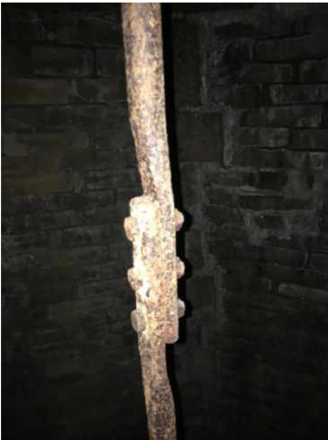
Holding down rod forged lap joint
