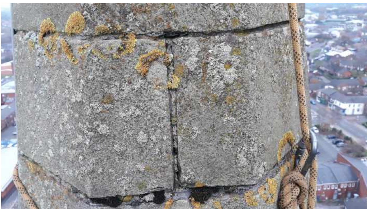
Pointing West face
