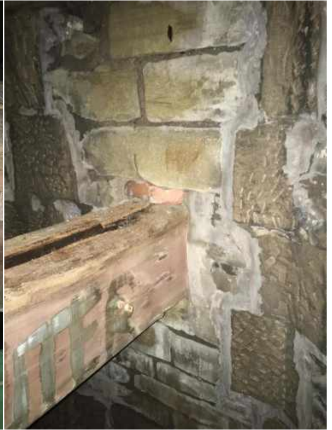
Wet rot to top of boards
