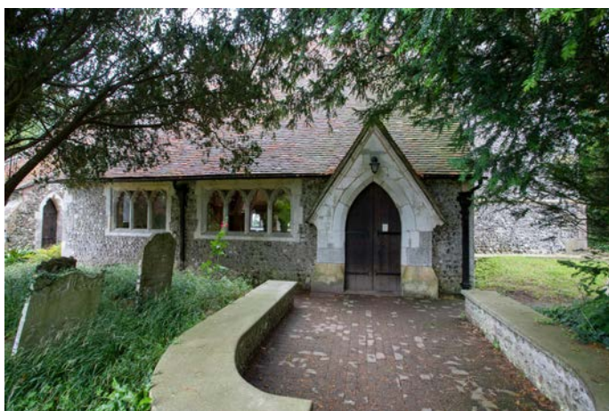
View of Woodyer's reconstructed north aisle and porch
