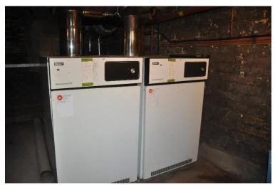
It was noted from the results of this flue gas analysis that while the flue gases are within the permitted limits there is more scope to adjust the burner to increase the efficiency of combustion. It is therefore recommended that the boiler engineer is requested to maximise the burner efficiencies during their next service visit.
