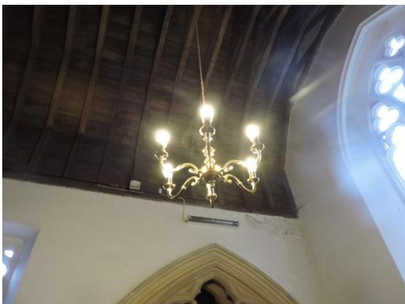
All the lighting within the church is currently efficient, low wattage compact fluorescent units. While these could be replaced for even lower wattage LED bulbs the saving is going to be rather low given the small hours of usage and therefore it is recommended that the conversion of the existing lighting to LED is made on replacement of the existing bulbs as the blow only.
