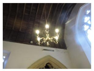
All the lighting within the church is currently efficient, low wattage compact fluorescent units. While these could be replaced for even lower wattage LED bulbs the saving is going to be rather low given the small hours of usage and therefore it is recommended that the conversion of the existing lighting to LED is made on replacement of the existing bulbs as the blow only.
