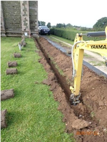
**Plate 26:** Excavation of the cable trench, from the north
