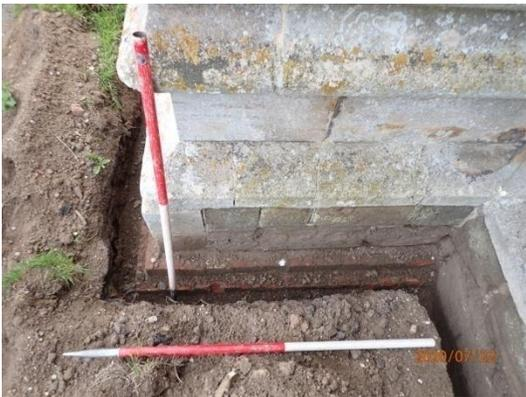
**Plate 10:** Exposed foundations of the north-western buttress of the West Tower, from the south
