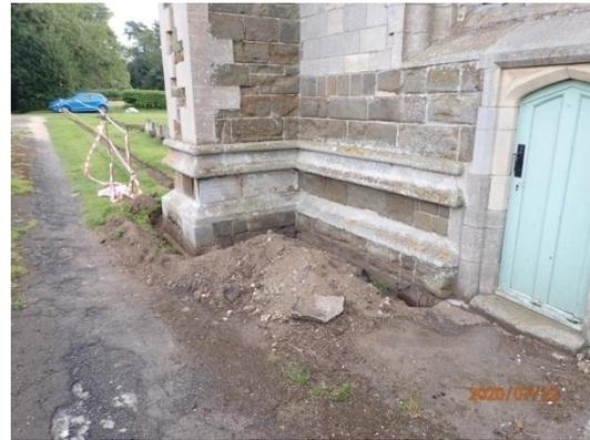
**Plate 5:** Hand excavated section of the cable trench around the north-western buttress of the West Tower & the West Tower, from the south
