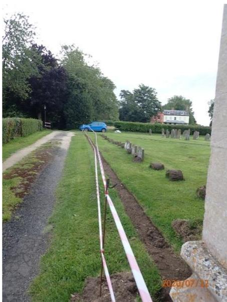
**Plate 3:** Set out section of cable trench, from the south
