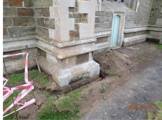
**Plate 4:** Hand excavated section of the cable trench around the north-western buttress of the West Tower, from the north-west
