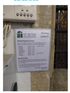
The heating is controlled via a domestic style 7 days programmer in the vestry. The notice next to this shows that the heating is set to come on for several hours each day.
