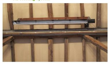
The hall is currently uses electric radiant heaters. These are not 100% efficient at converting electricity to heat since they produce some light, but are efficient. Should they require replacement, radiant far infrared panels are recommended (these do not produce any visible radiation).
