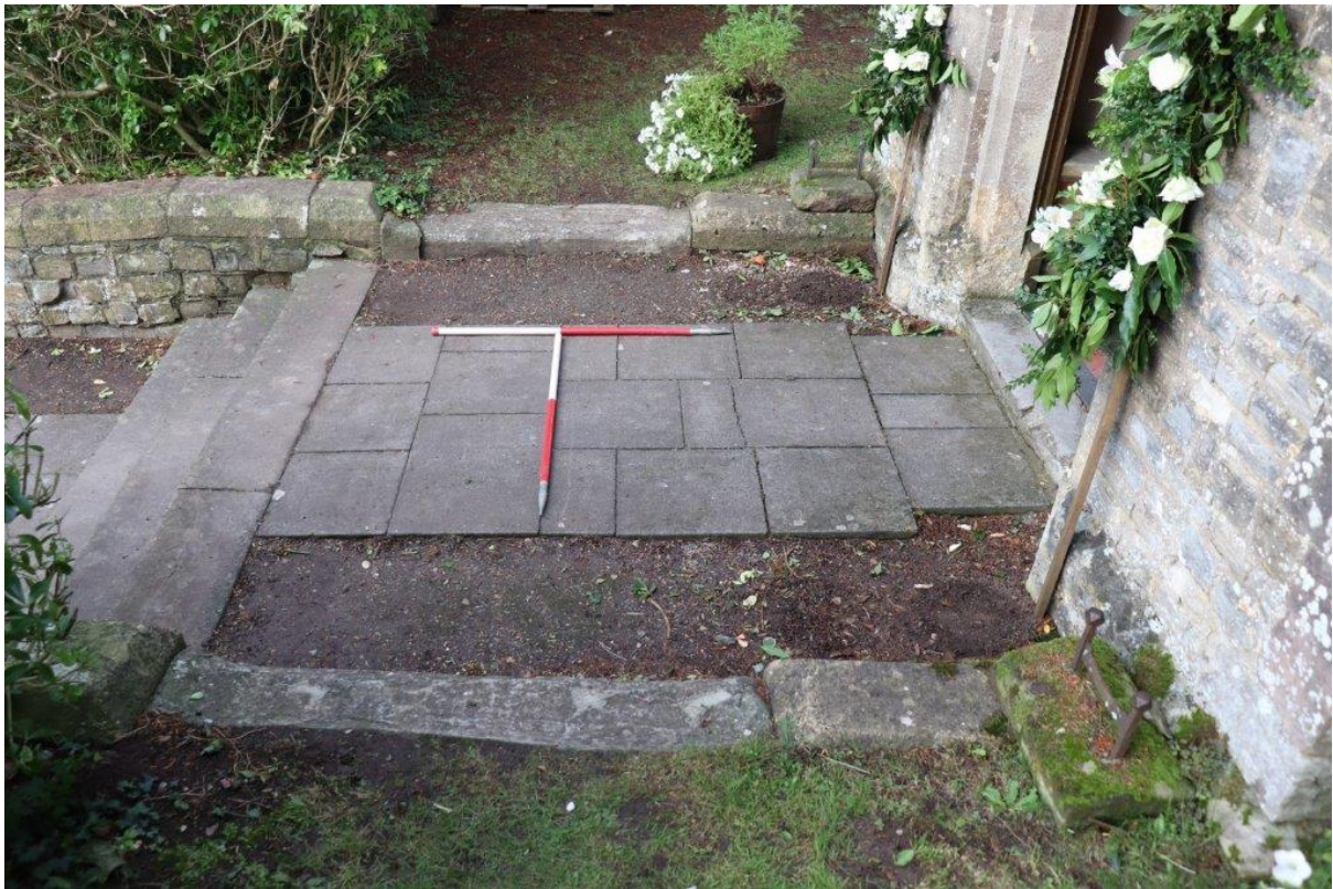
Plate 7: Concrete paving slab path and loose soil. 2 x 1m scales. View west
