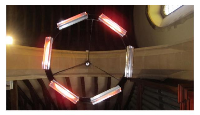
At Marden, if similar chandelier heaters were suspended from the midpoints of the six arches in the nave, they would probably have to be of larger diameter than above, possibly with eight elements each. The outside portions of the aisle seating would be furthest from the source of heat: these might require some additional ceiling mounted white rectangular far infrared panels.
