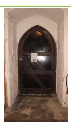
Daylight is visible under the Lady Chapel door to the left, and around the top right frame of that in the image on the right. A large gap was observed under the tower west door.
