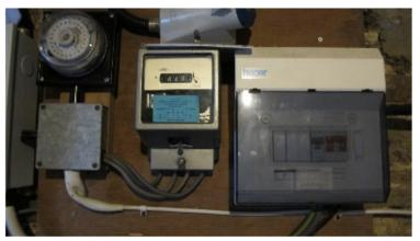
The electricity meter (left) is AMR connected and as such energy profile for the annual usage should be possible. There is a submeter to record the floodlighting consumption (right).
