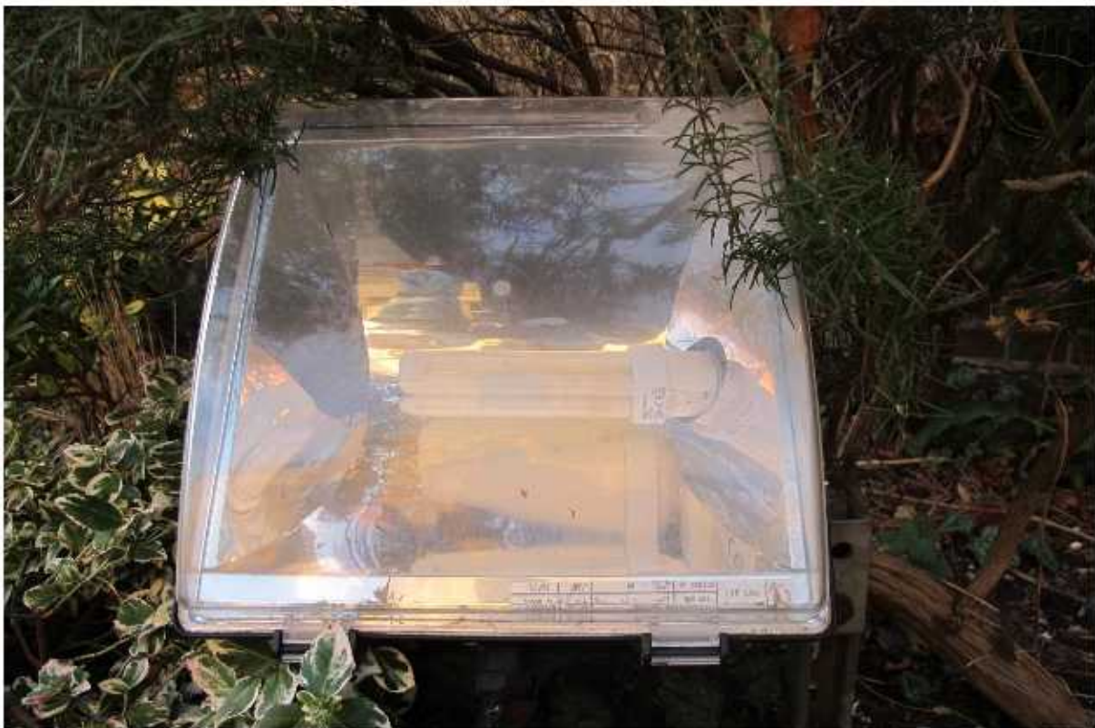
42W CFL floodlight
