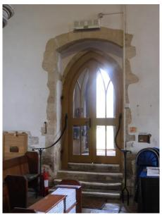
In order to achieve the sense of a 'warm welcome' into the church an over door air heater could be provided. This would also help to provide warmth to the rear of the church up to and include the font. Such an over door unit should be sized to cover the whole width of the door and it is suggested the BN Thermic 860 model would be quite suitable.
