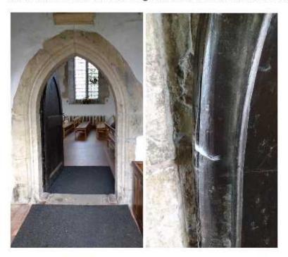
The porch door has a leather strip which closes against the stonework. This should be kept maintained and effective. If the space is too large for a flap to keep airtight, rolling a long strip of leather around some fabric / foam / horsehair (something soft, compressible and elastic) and pinning it to the door with brass tacks would be effective.
