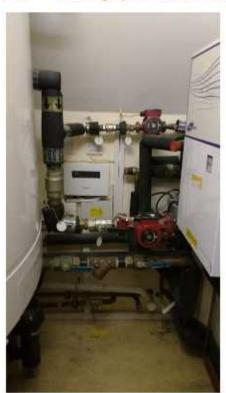
The church currently uses two Worcester Logamax Plus 50kW gas boilers installed in 2019, one to heat the church and one the offices. This is reported to work well and provides adequate thermal comfort into the church. Given that the system is successful and not overly wasteful of energy we would recommend that this system is continued with and consideration is given to the following improvements.
