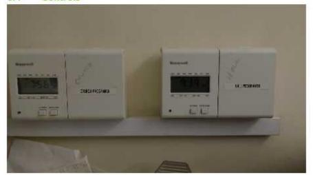
Boiler timer controls are located in the boiler room on the second floor. It is suggested that a simple set of "how to" instructions are laminated and displayed adjacent to the controls which also indicate who has permission and who should be informed of changes and problems.
