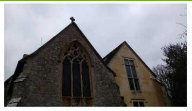
The office building roof offers an area of around 10m<sup>2</sup>. This could generate 0.15kWpeak/m<sup>2</sup> giving a 1.5kWpeak system. A 1kWpeak system can generate 1000kWh annually in Kent, although due to the proximity of the chancel roof an over shading factor should be applied to give a total annual generation of 1350kWh. This is in the smaller than the church's annual electricity use of 5200kWh.
