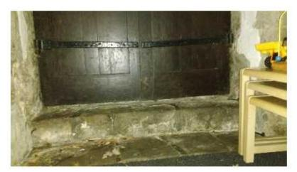
If the tower door (above) is rarely used it should be made airtight.
