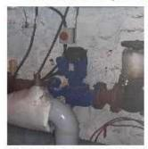
The existing pumps within the building are fixed speed units meaning that they are either running at full power or they are off. In varying conditions, the pumps and fan motors will only need to operate at part power and can consume less energy in doing so.
