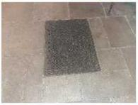
The main heat emitters to the church nave is via floor grills. Looking through them, the pipes are very dirty and covered in a
