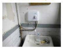
There are a number of electric point of use water heater in the toilet and vestry to provide hot water for hand washing. This only needs to heat the water to the required temperature when the building is in occupation but at the moment this heater is directly wired in without any form of time control and therefore maintains its set temperature 24/7.
