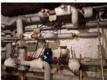
The pipework within the plant room has the majority of its straight lengths insulated and a number of the more complex shaped pipework fittings, such as valves, have been insulated. However, some of the specialist jackets have been removed and not replaced. These exposed areas of pipework contribute significantly to wasted heat loss from the system and make the plant room unnecessarily warm. The exposed hot surfaces also
