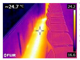
Within the church, the pipework has been housed within wooden boxing which will reduce the ability to convect heat into the space where it is required. It is suggested that the boxing is considered to be removed to allow greater heat distribution into the main body of the church as the pipework is essentially acting as a radiator.
