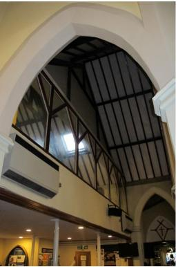
Electric heat means this part of the building can be heated by 100% renewable energy if the church signs up to such a tariff. On average, grid electricity currently emits more  $CO_2$  than gas, it's footprint is rapidly falling as further wind generation capacity is added, replacing coal. The comparison of non-renewable "brown" tariffs is 0.25kg  $CO_2$  per kWh for electricity and 0.18kg  $CO_2$  per kWh for gas.
