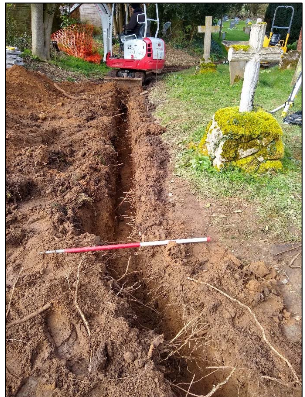
Plate 3. Service trench. Looking west, 1m scale
