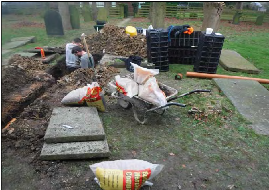
Plate 2. Working shot showing excavation of the soakaway, facing northeast
