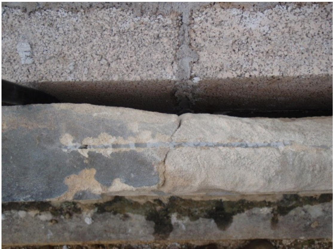
Detail showing stainless steel reinforcement/repair.
