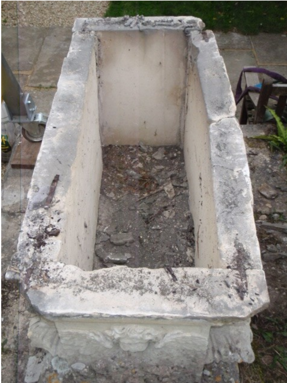
The lid was removed to enable replacement of rusted iron cramps.
