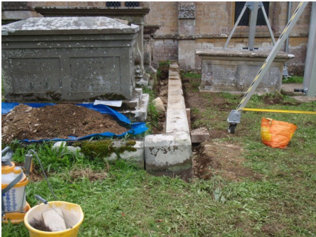
The north-west plinth stone after repositioning.
