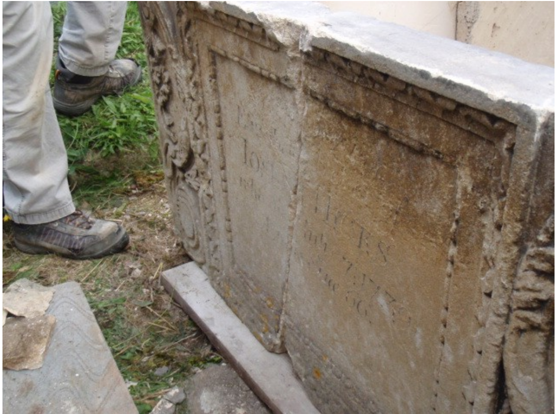
The north side panel pieces repositioned using polyester resin.
