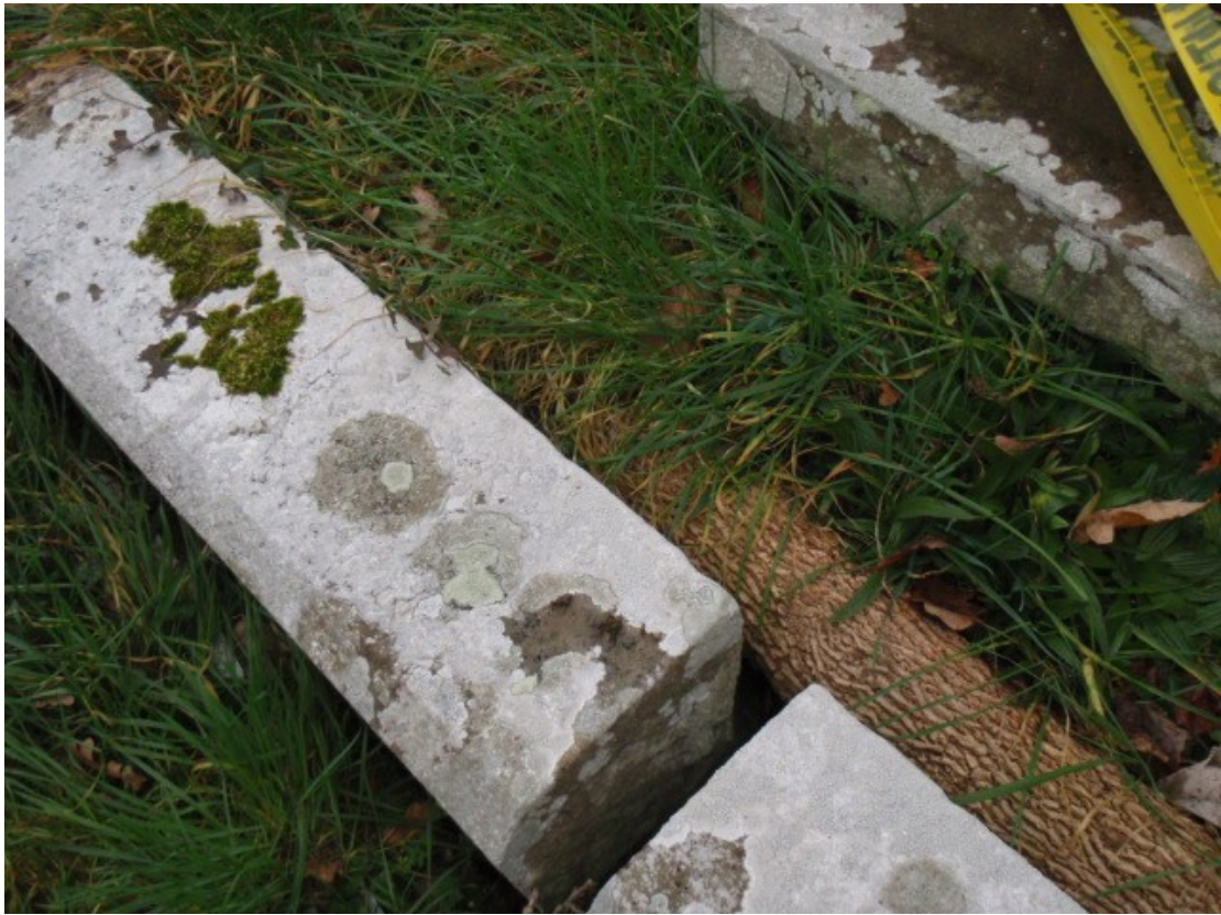
The gap, exposing the interior of the burial chamber, temporarily filled by a log.
