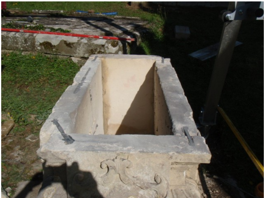
Rusted iron cramps were replaced by stainless steel ones.
