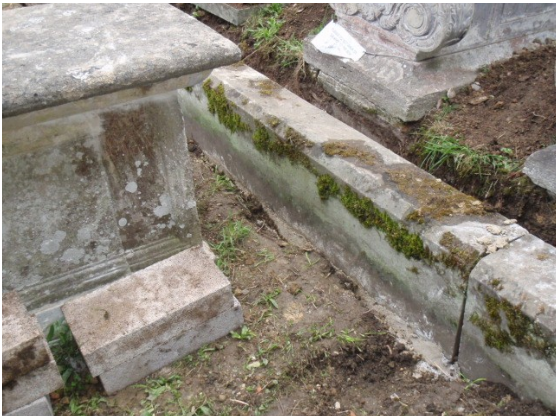
The stones rebbeded on lime concrete.
