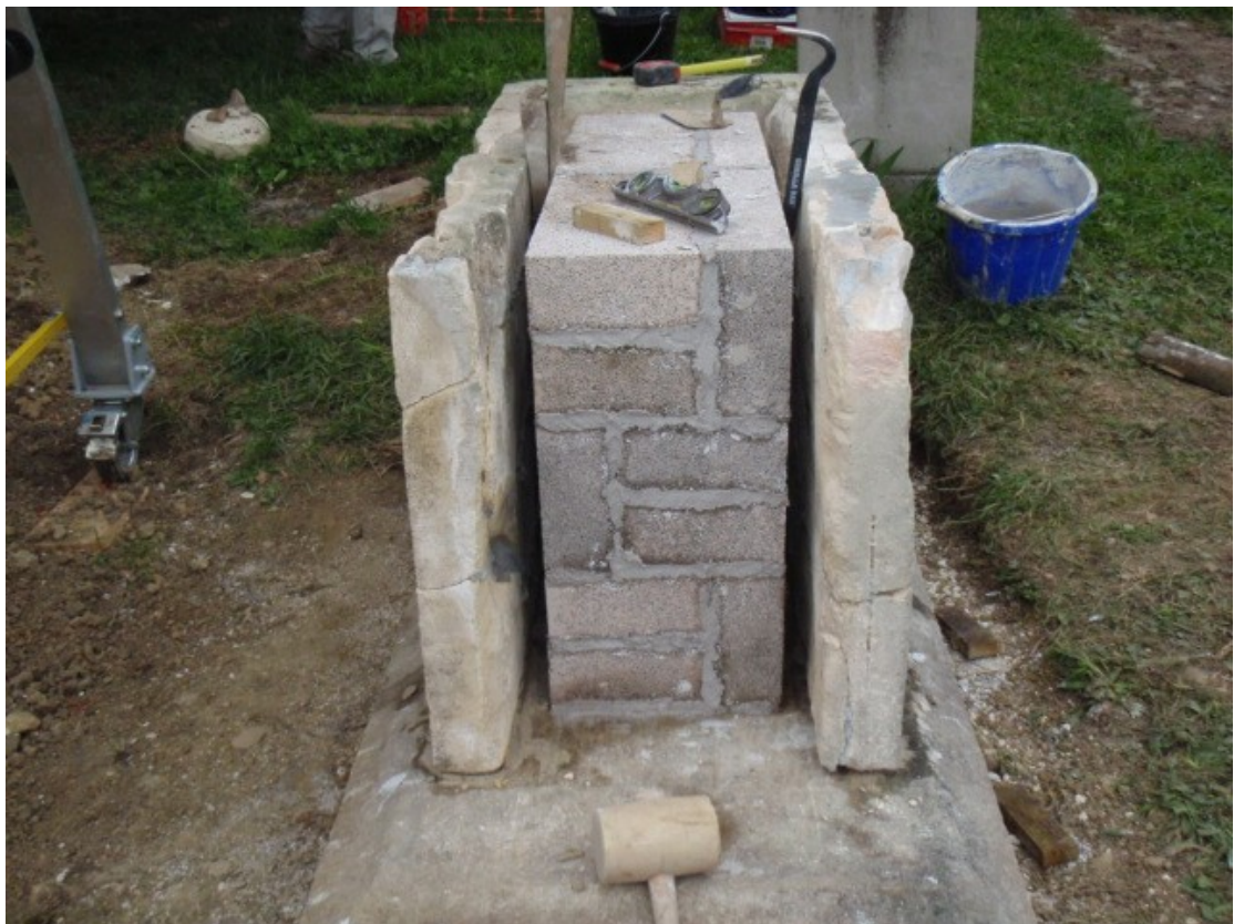
The repaired side and end panels were rebuilt around a blockwork core.
