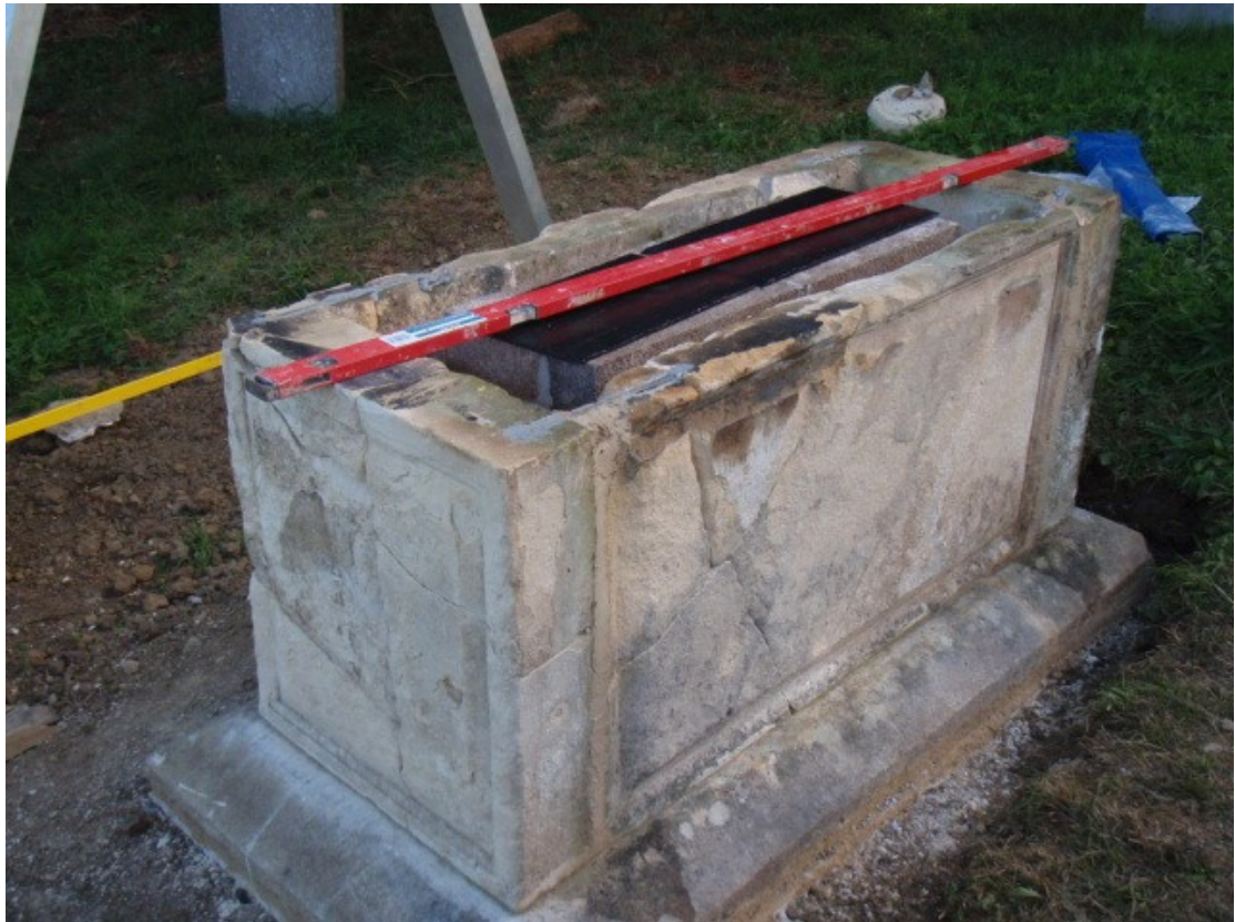
Slates were added to raise the top of the core above the sides.
