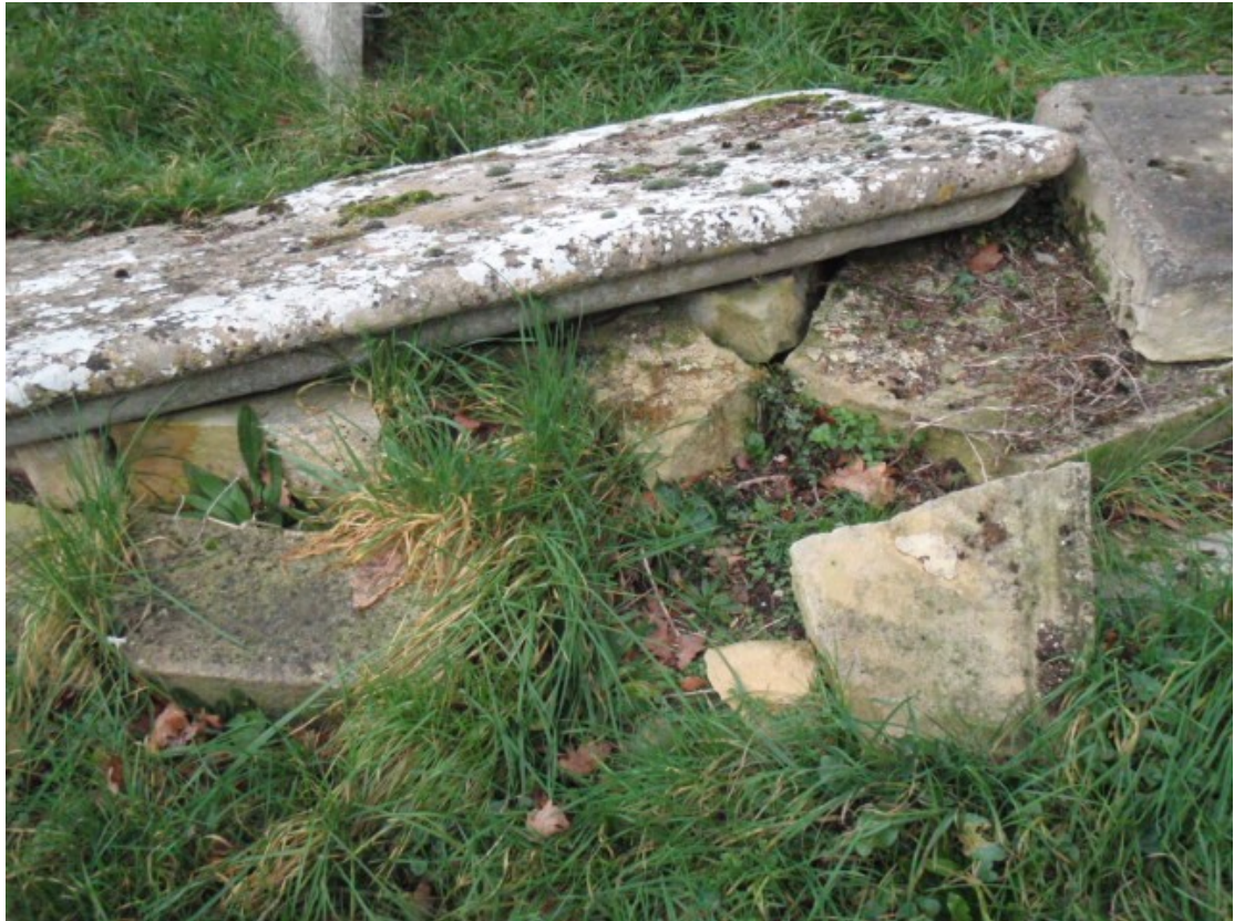
Broken pieces of the north and south side panels lie under the lid.
