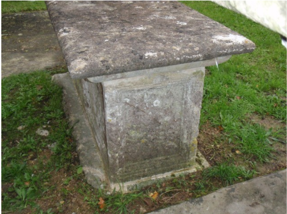
East end after conservation.
