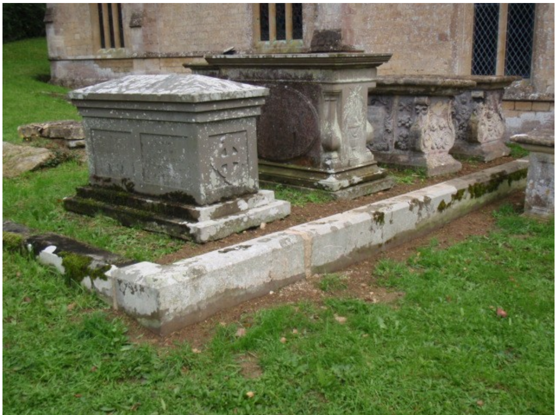
The completed works, viewed from the NW.
