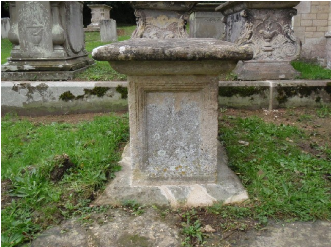
West end after conservation.
