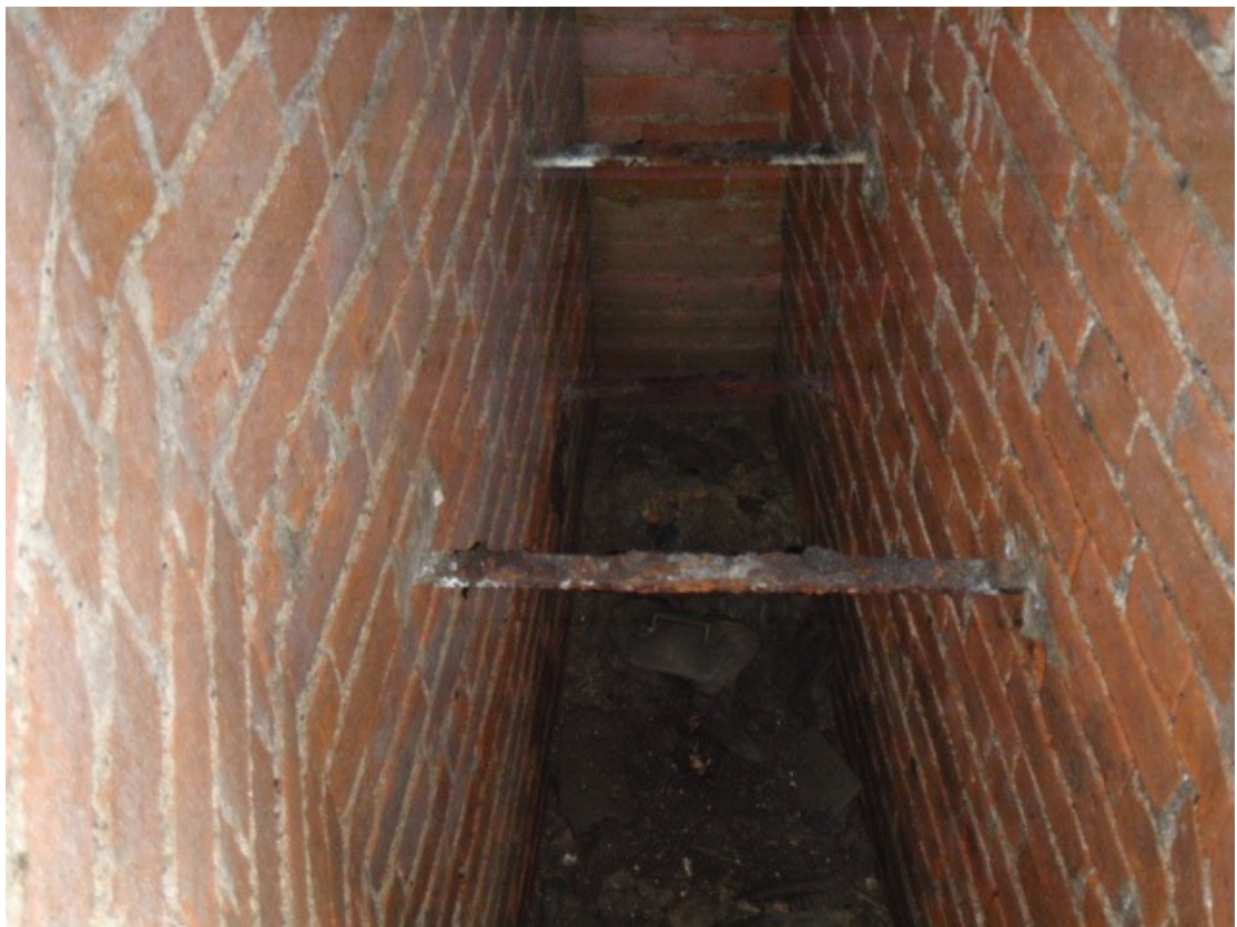
The brick-lined shaft beneath the John Marbett 1879 monument.
