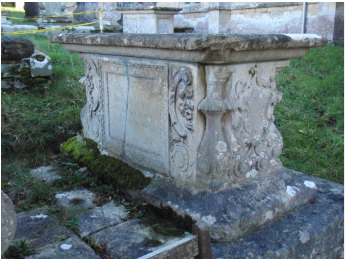
Note previous repairs carried out using Portland cement.
