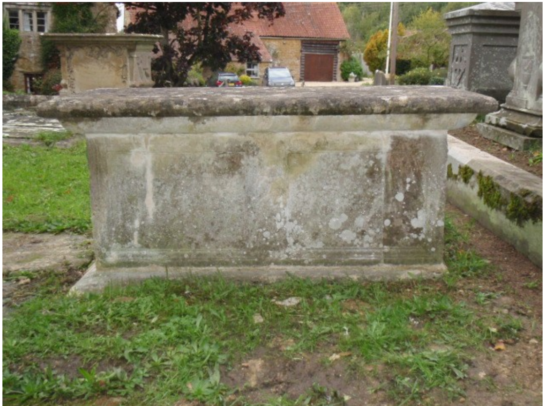
South side after conservation.
