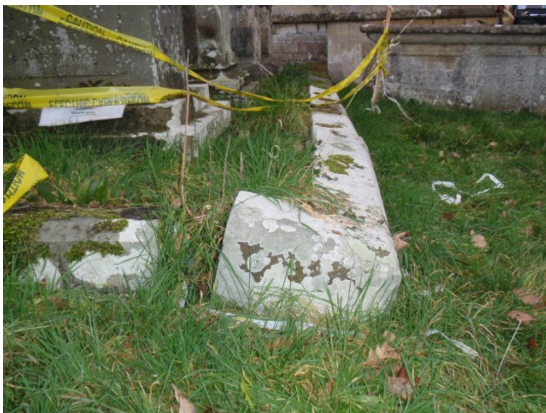
The north-west plinth stone, rotated due to subsidence.
