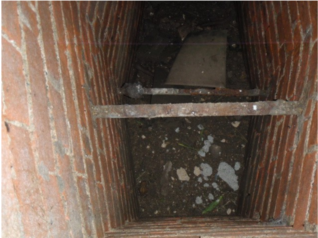
The west (head) end of the shaft.
