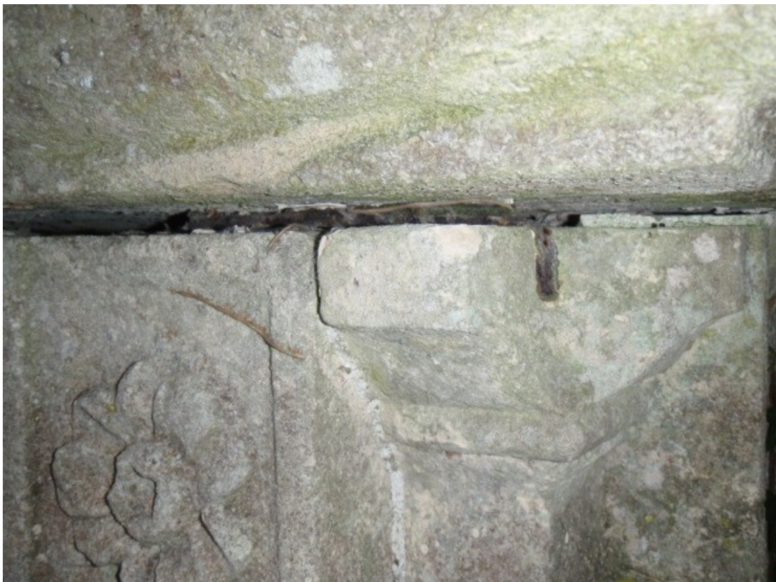
A similar cramp at the south-east corner. This one has also broken off the corner
