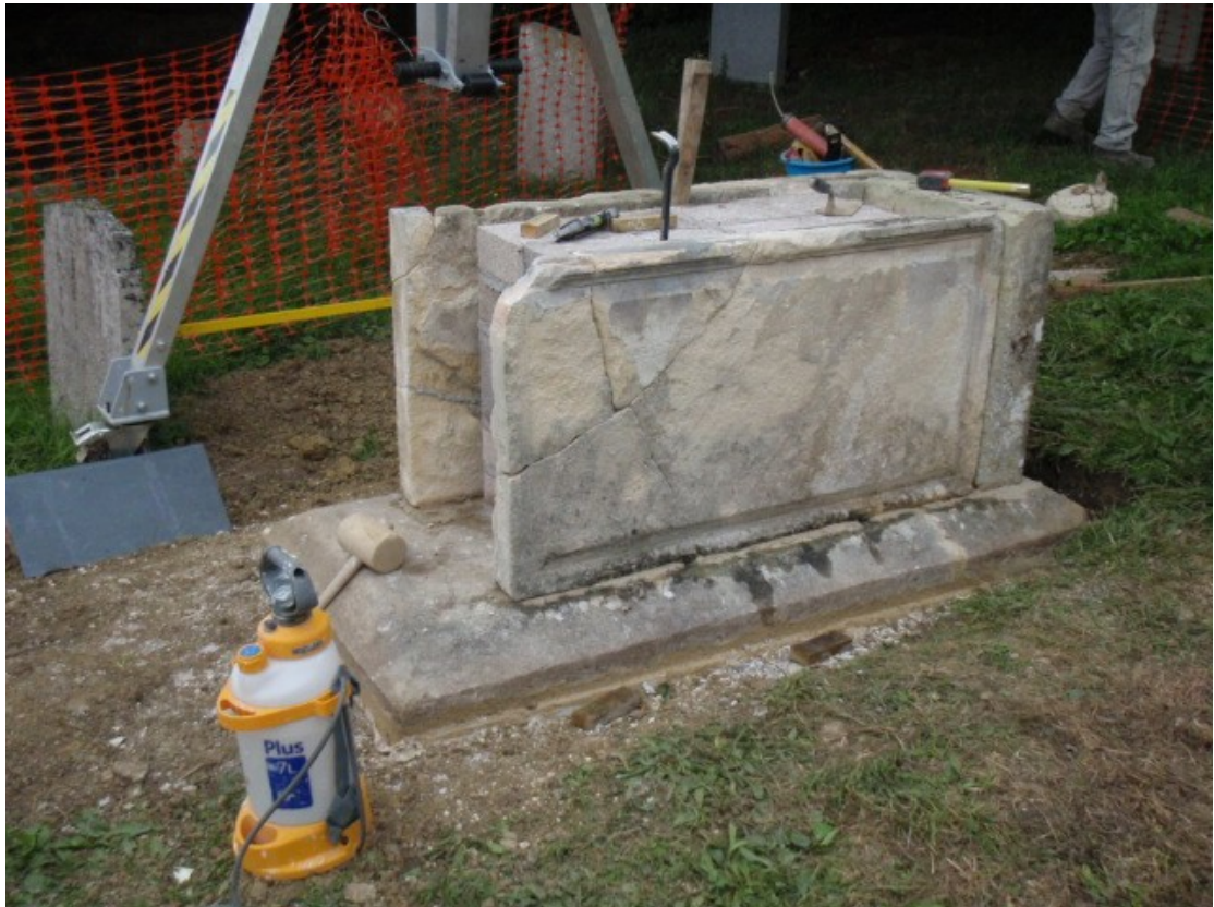
The repaired side and end panels were rebuilt around a blockwork core.
