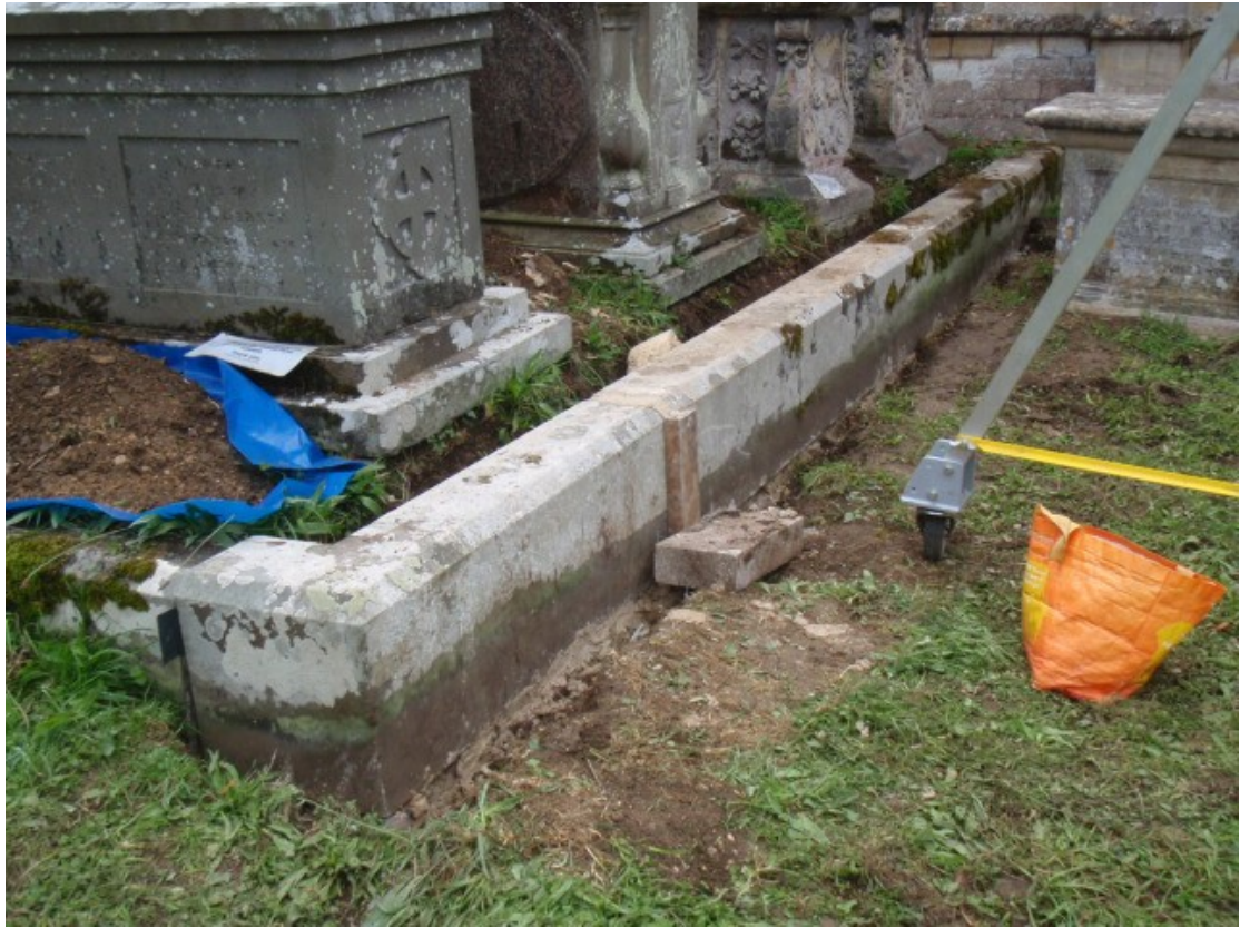
The stones rebbeded on lime concrete.
