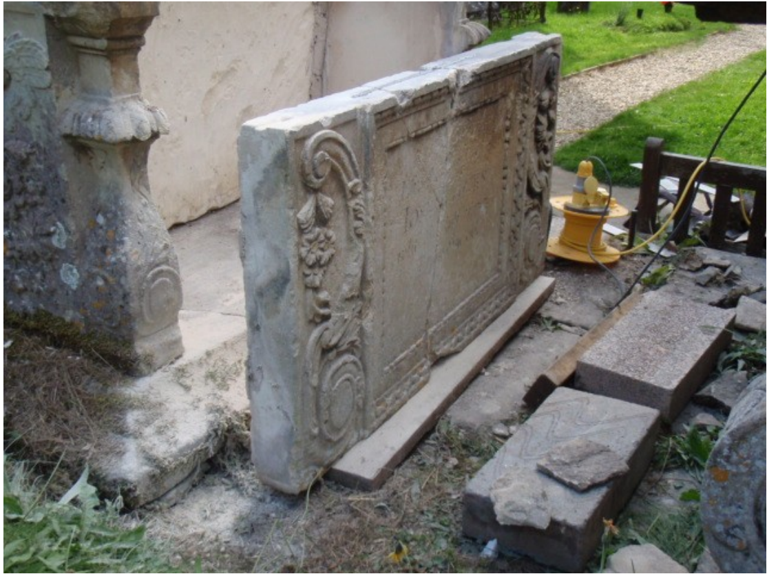
The repaired panel prior to reinstatement.
