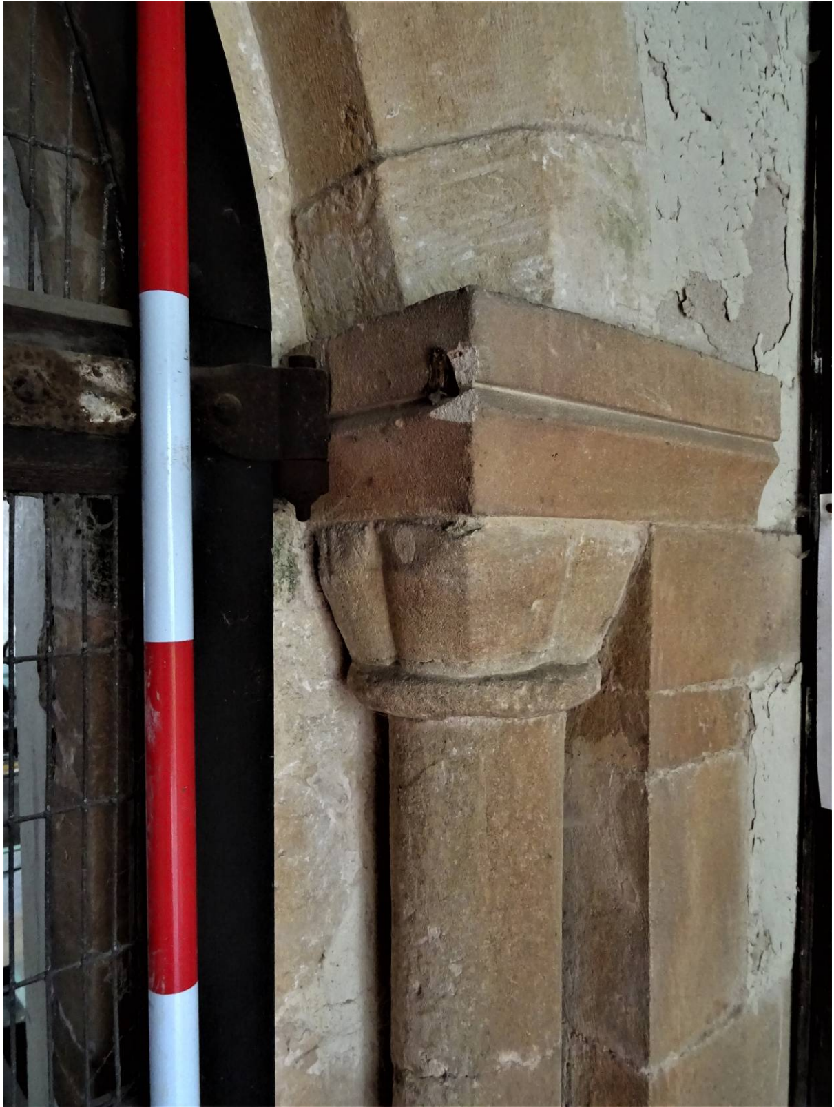
Plate 7. Detail of the eastern moulded column
