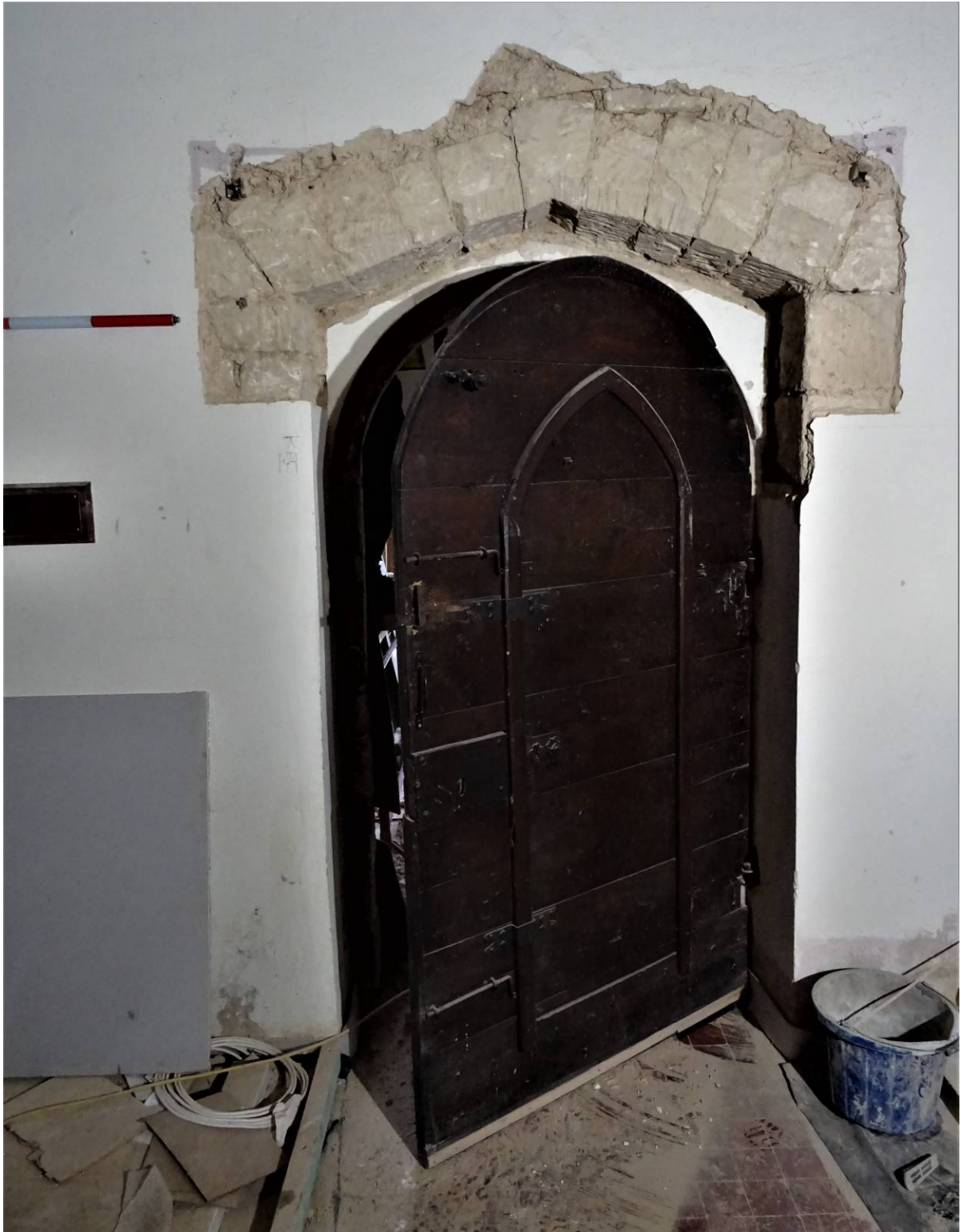
Plate 14. Exposed perpendicular arch, exposed during render removal
