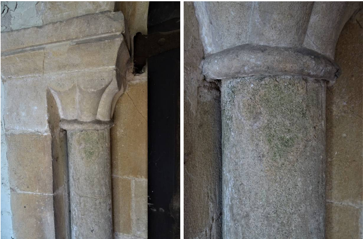
Plate 5. Upper section of a decorative moulded column flanking the western side of the door
