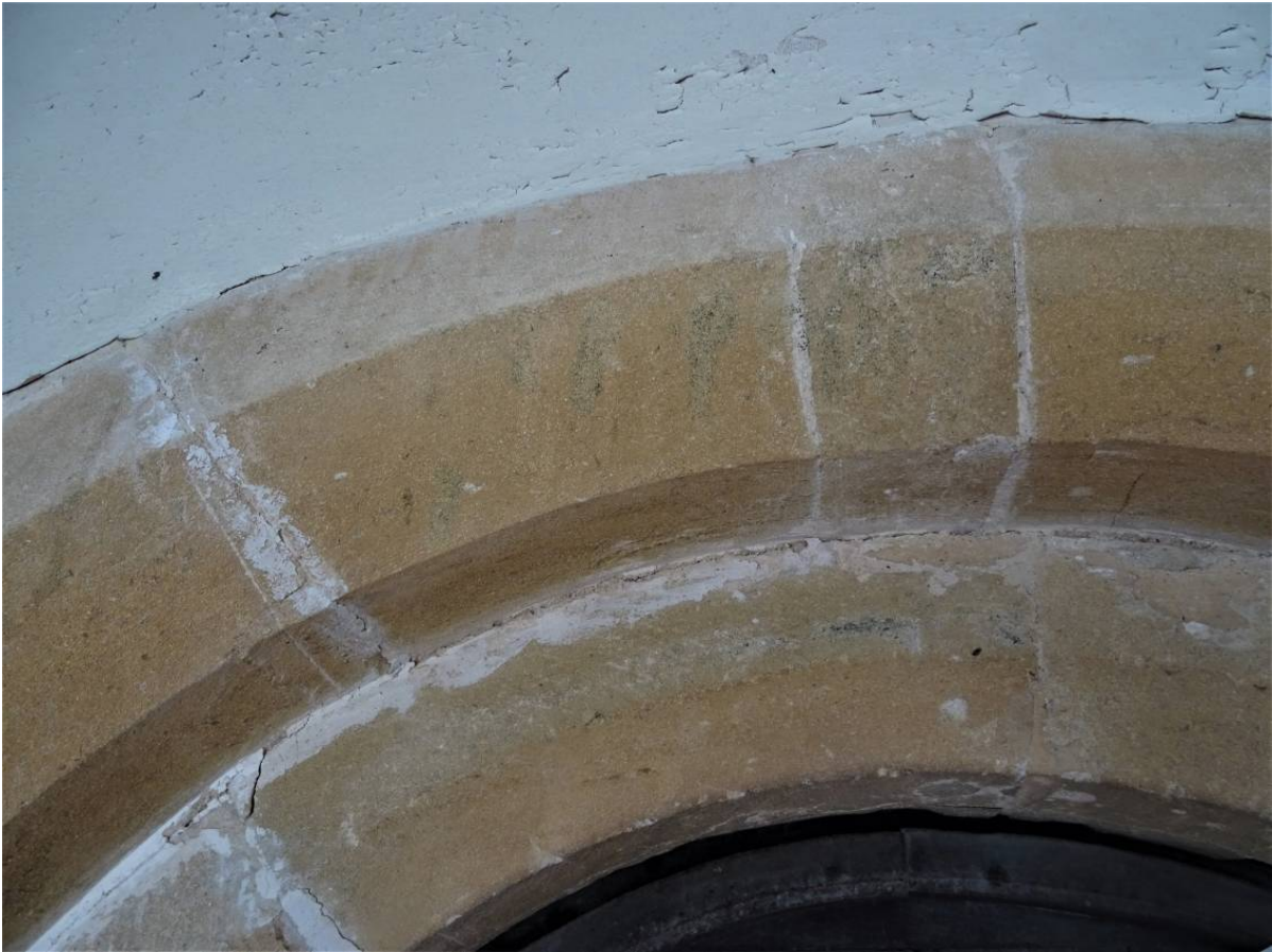
Plate 4. Detail of the dressed stone forming the arch
