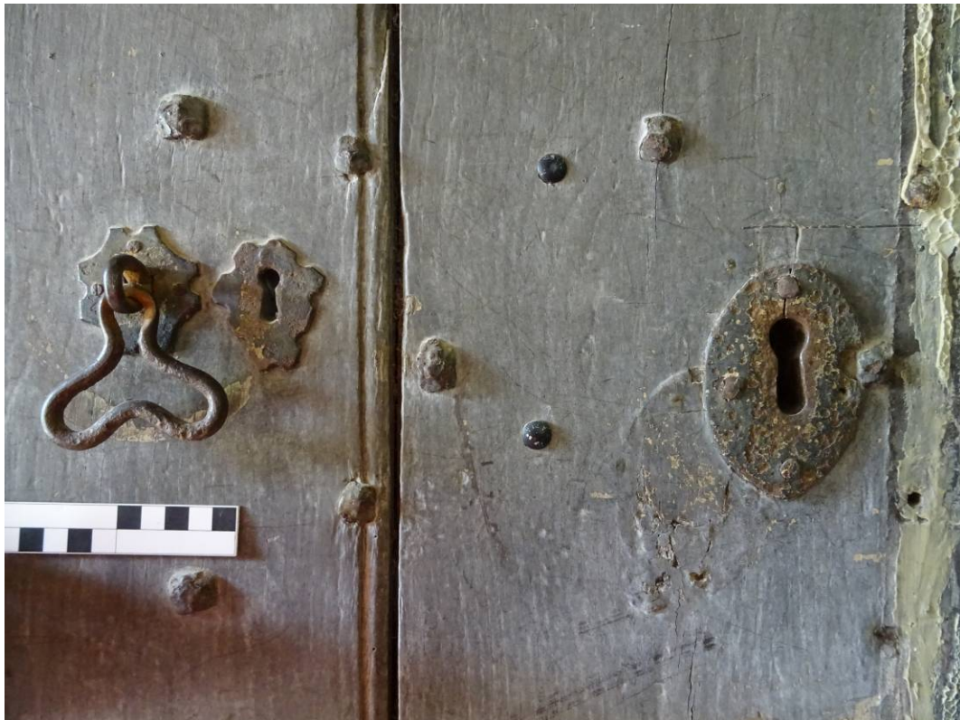
Plate 12. Mid- to Late 17 th century drop handle and lock-plates incorporated into the door
