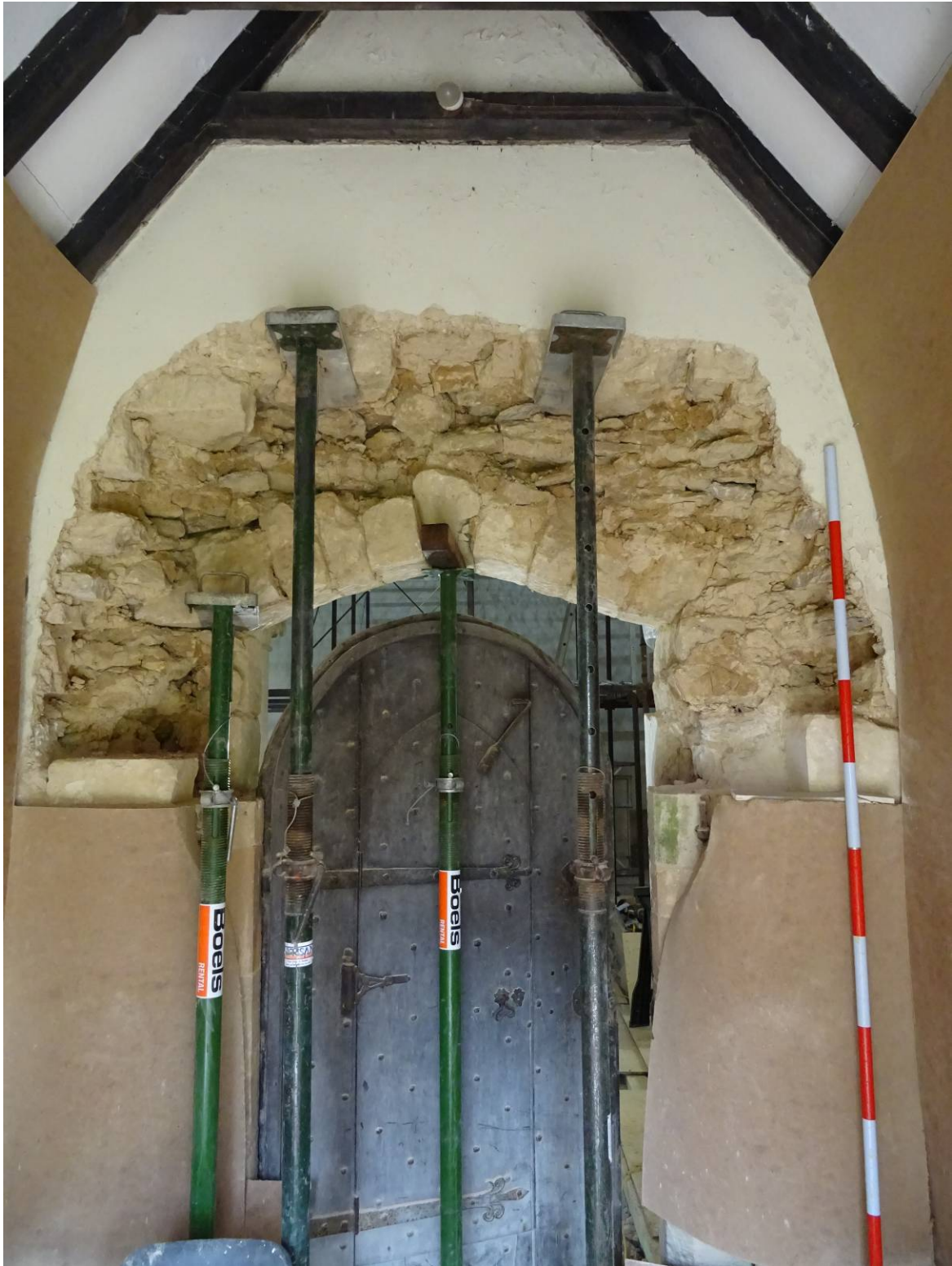
Plate 17. Removal of render to expose rubble surface and perpendicular pseudo-four-centred arch
