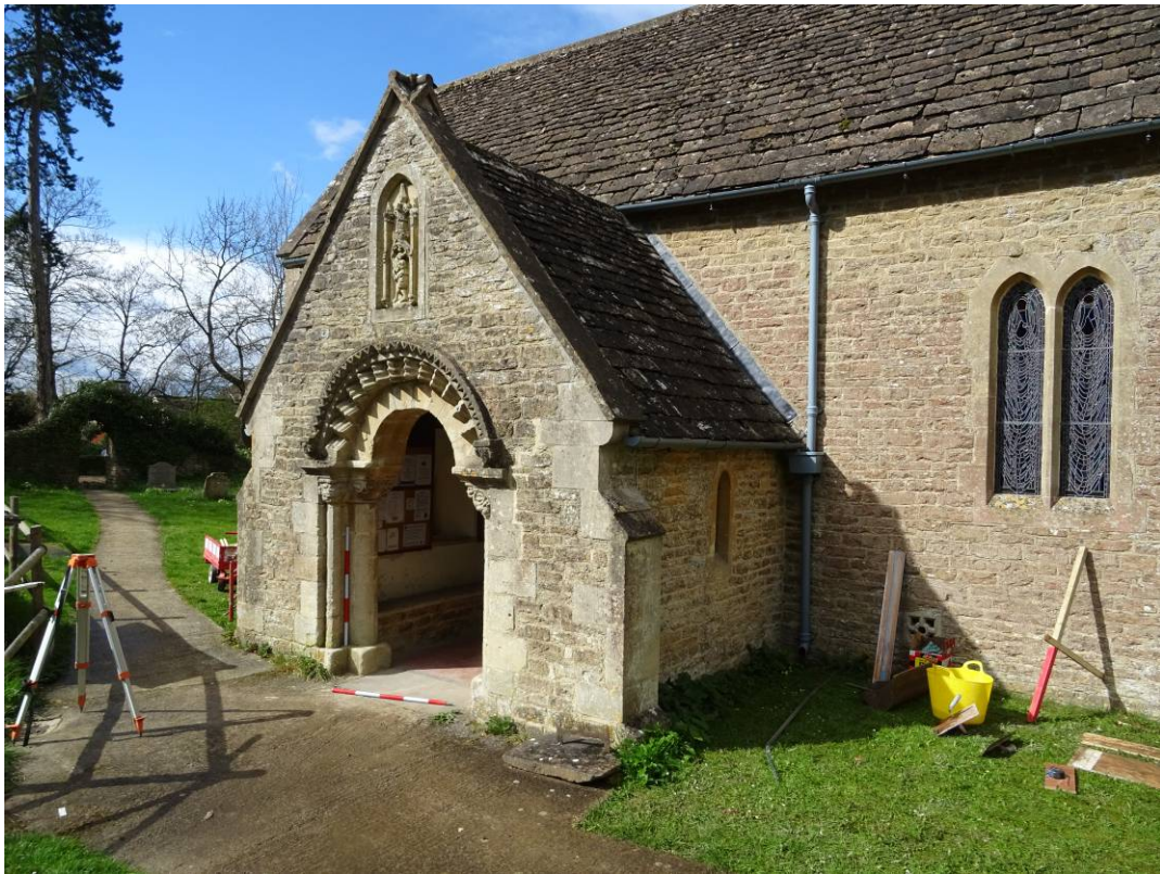
Plate 1. South porch dating to the 19 th century abuts the medieval fabric of the southern elevation
