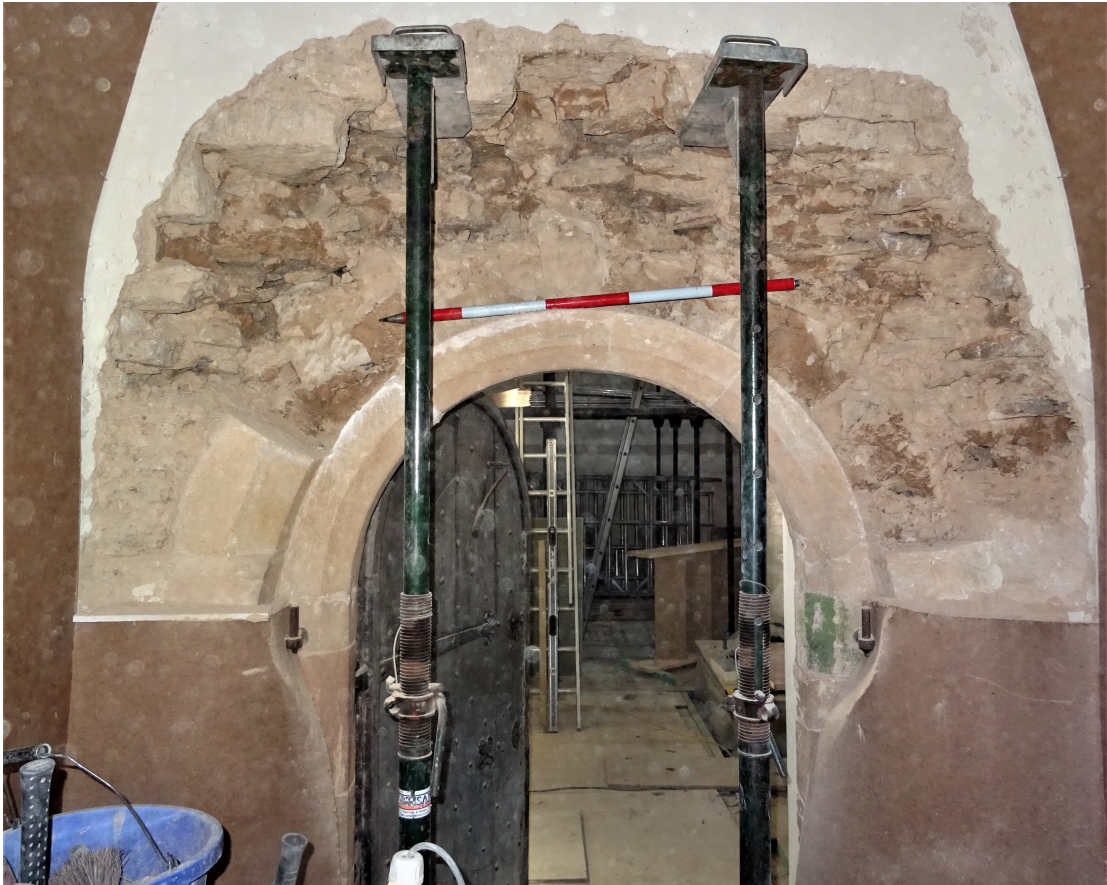
Plate 15. Removed render exposing the rubble stonework, view from the porch
