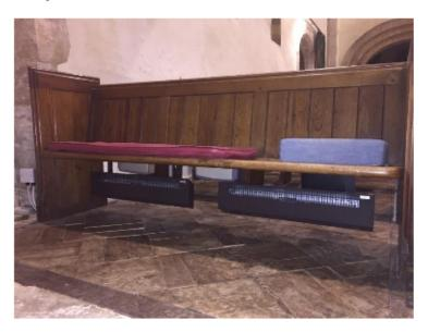
An alternative design which is available in a variety of lengths (and hence outputs) is the "Cooltouch" fabric covered radiant under pew heater. https://www.cooltouchheaters.co.uk/
