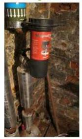
The boiler does not appear to be fitted with a magnetic particle filter as illustrated below. This apparatus catches any rust or metal particles and prevents them being deposited on the boiler heat exchanger. One should be installed if it is planned to continue using this heating system long term. Corrosion inhibitor should be added to the system when your boilers are serviced annually.
