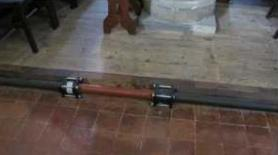
As discussed, there are places where the redundant surface pipework constitutes a trip hazard and should be removed.
