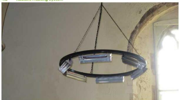
Heating is provided by five overhead rings of six radiant heaters in the nave / aisle area and a further two in the chancel which are rarely used. These are arranged to appear as a chandelier; thus the glowing effect of the traditional visible/IR radiant heaters is considered acceptable. Located level with the column capitals, they appear visually compatible with the surroundings.
