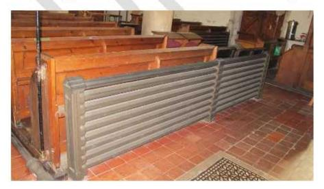
The previous heating system was run from an oil fired boiler, giving a high rate of CO<sub>2</sub> production per kWh of heat and long warm up times.
