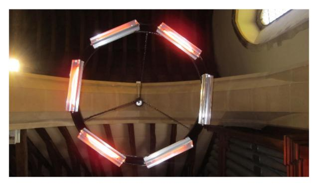
Ten chandeliers with 6 elements each installed up to the choir stalls area would provide 60kW of heat at a capital cost of around £30,000.
