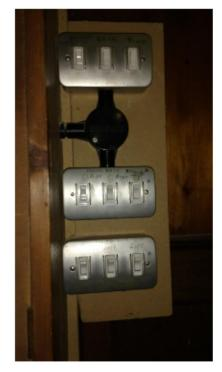
The existing lighting control panel is poorly labelled. It would benefit from a laminated colour coded diagram as the current markings will wear off with use.
