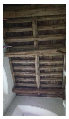
Much of the ceiling of the aisles is comprised of closely spaced beams with no location for radiant panels between the beams. This indicates either mounting radiant panels on the walls, or using chandelier type heating.
