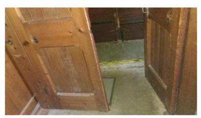
There are a number of external timber doors in the building. These should be kept maintained and draught proofed where possible to prevent cold air from coming into the church around the side and base of these doors.
