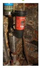
The boiler did not appear to be fitted with a magnetic particle filter as illustrated below. This apparatus catches any rust or metal particles and prevents them being deposited on the boiler heat exchanger. They should be installed if it is planned to continue using the water heating systems long term. Corrosion inhibitor should also be added to the system when your boilers are serviced annually.
