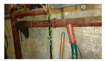
It is recommended that these areas of exposed pipework and fittings are insulated with bespoke made flexible insulation jackets. These wrap around the various elements but can be removed and then replaced for any servicing activities.
