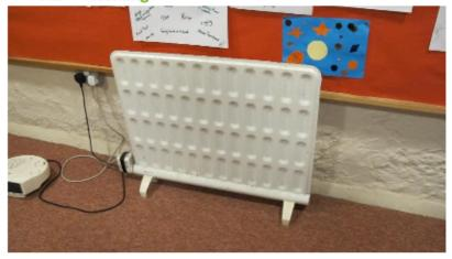
This oil filled radiator has a long heat up time and will be ineffective at heating the space.
