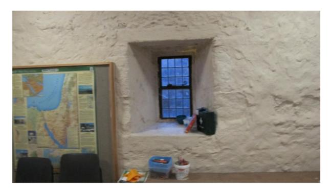
Secondary double glazing can be achieved by using "seasonal" double glazing plastic film (which will also reveal if there is a draught through the window). Any gaps can be filled with black plasticine, which is easily removable. Permanent secondary glazing would require faculty permission given the listed status of the building.
