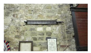
The ringing chamber would benefit from more efficient far infrared panel heaters which could replace radiant bar heaters.
