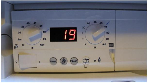
The water temperature is set to 70°C, which may be too high for it to act as a condensing boiler. It is unclear whether the boiler circuit includes the choir vestry radiators and the underfloor heating, or if the UFH has a separate heat exchanged on the circuit.
