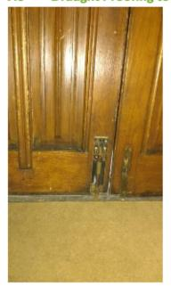
The western pair of doors has a gap between the two doors when they close which is big enough to admit a large amount of air when it is windy. This will be a constant source of heat loss throughout the heating season, in fact at all times when the external temperature is colder than the internal temperature in the church.
