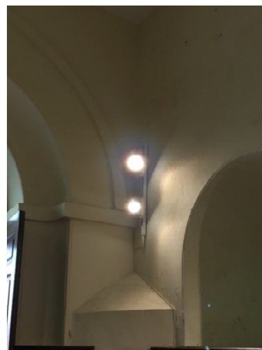
Photograph 7: LED Hanging Lamps
