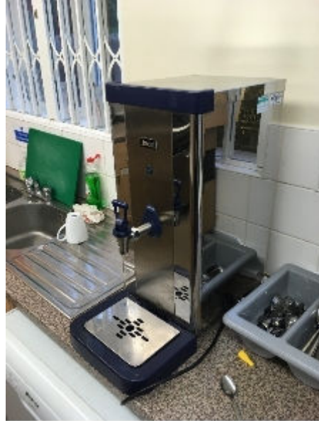
Photograph 6 and 7: Electric Water Heaters
