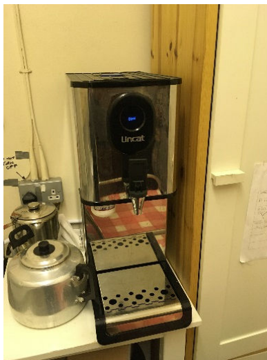
Photographs 6 & 7: Electric Water Heaters
