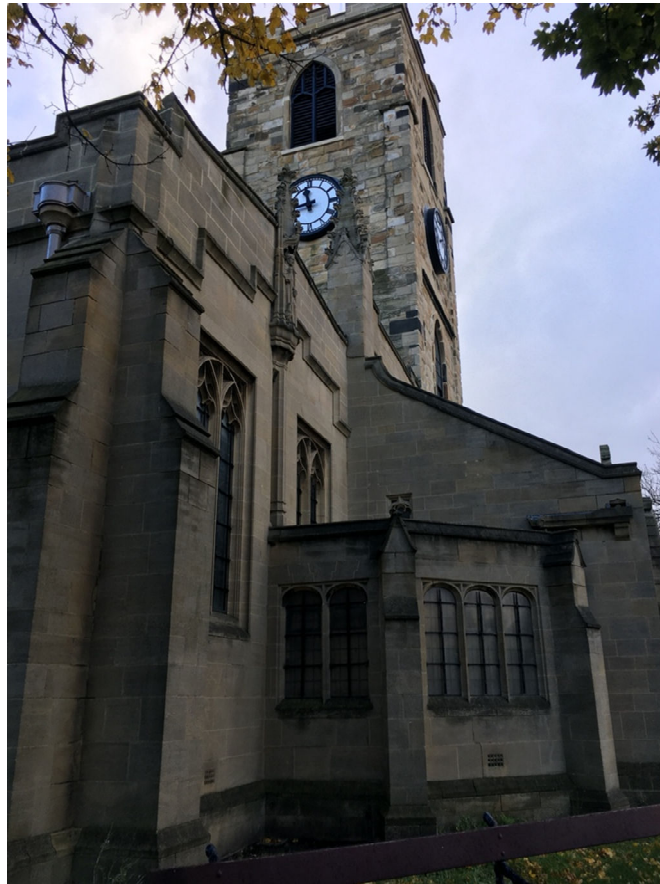
Photograph 1: Minister Church of St. Michael & All Angels External View
