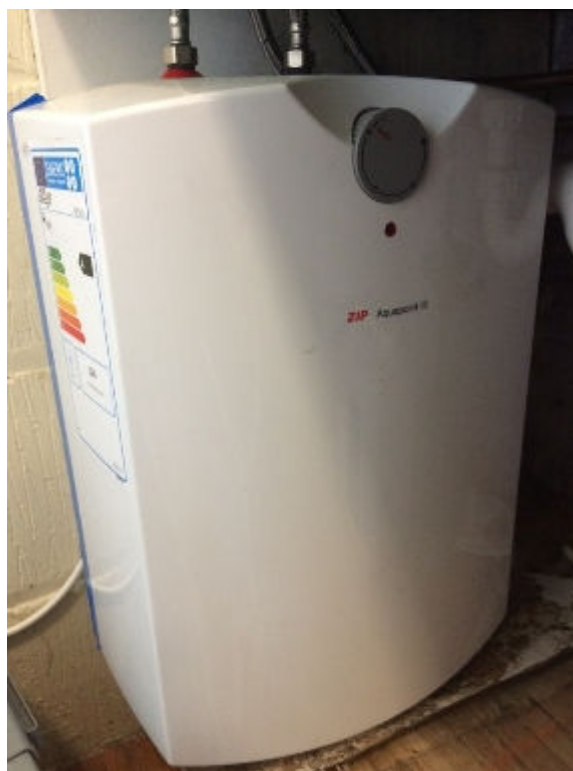
Photograph 6 & 7: Electric Point-of-Use Water Heater and Aquapoint Water Heater
