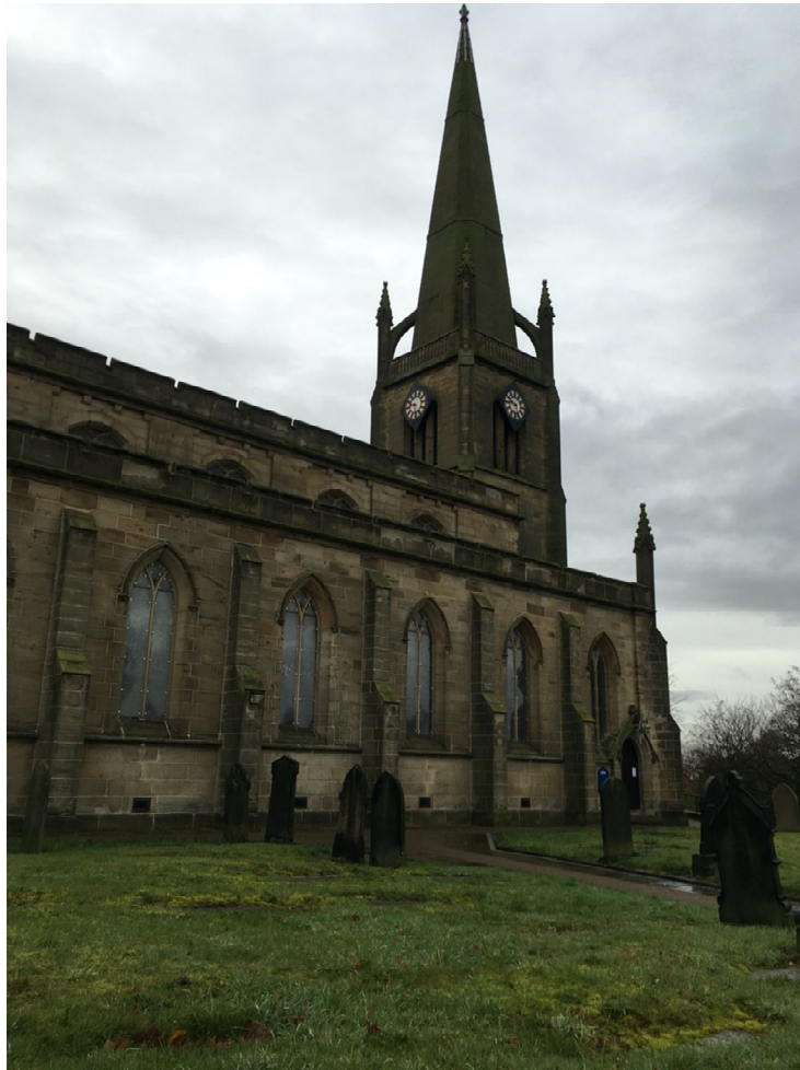
Photograph 1: St. George's Church External View
