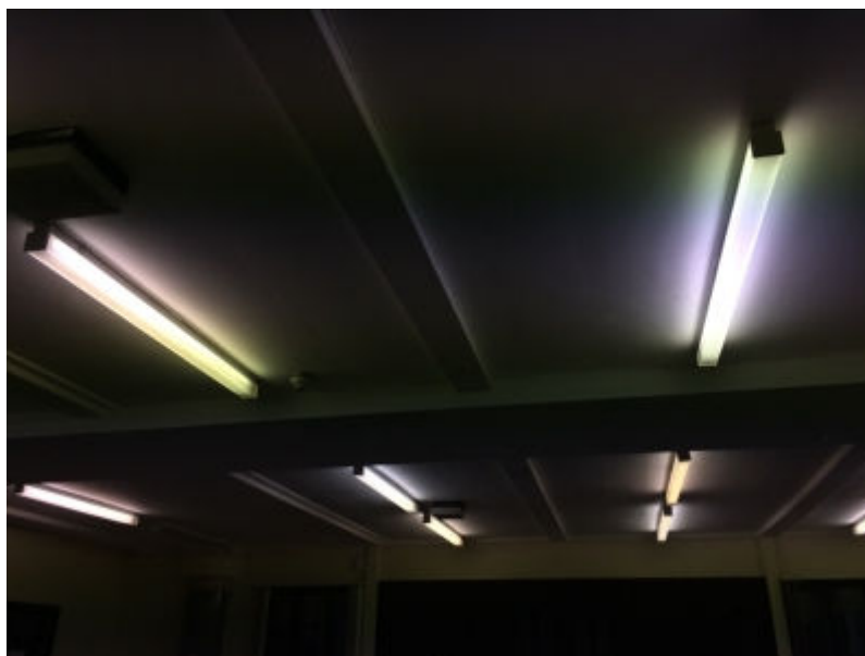
Photographs 10: Church Hall Light Fittings
