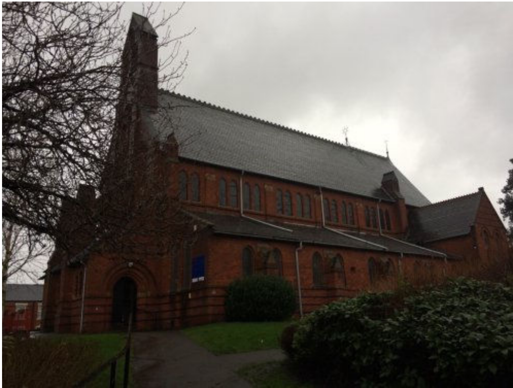
Photograph 1: Holy Trinity Church External View
