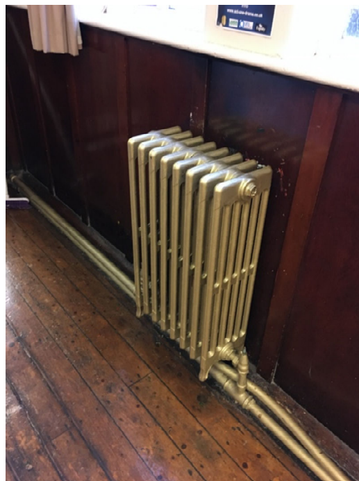
Photograph 4: Church Hall Iron Radiators
