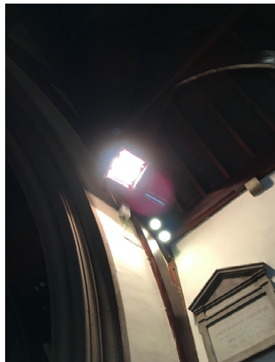
Photographs 2 & 3: Gas Radiant Heating System & Electric Wall Heater
