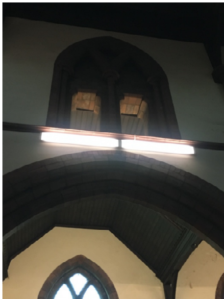
Photographs 6 & 7: Twin Fluorescent Tubes and Halogen Floodlights
