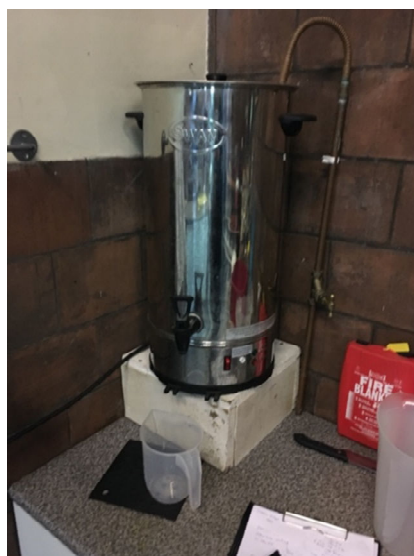
Photograph 5: Electric Point of Use Water Heater
