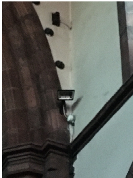
Photographs 6 & 7: Twin Fluorescent Tubes and Halogen Floodlights
